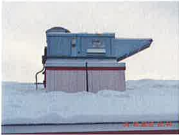
Roof exhaust and air intake
