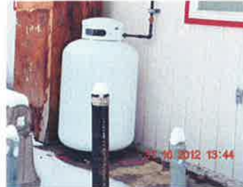
Propane tank for range and make-up air heater
