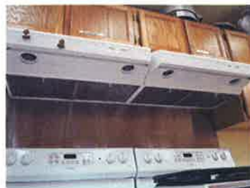
Non-vented ventilation system before renovation
