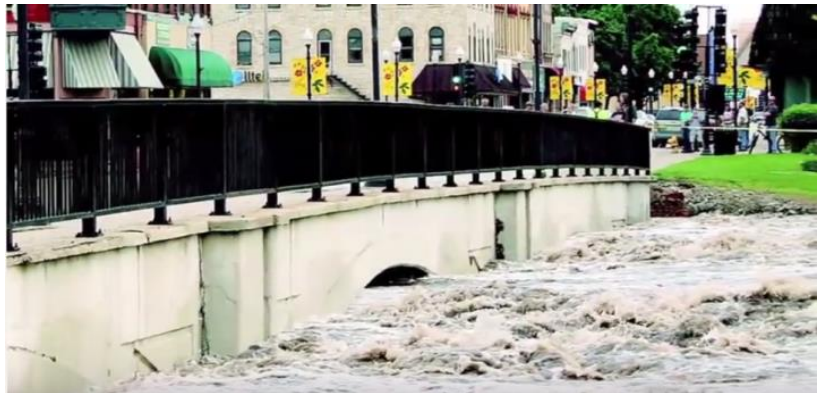
Main Street Bridge During 2008 Flood
