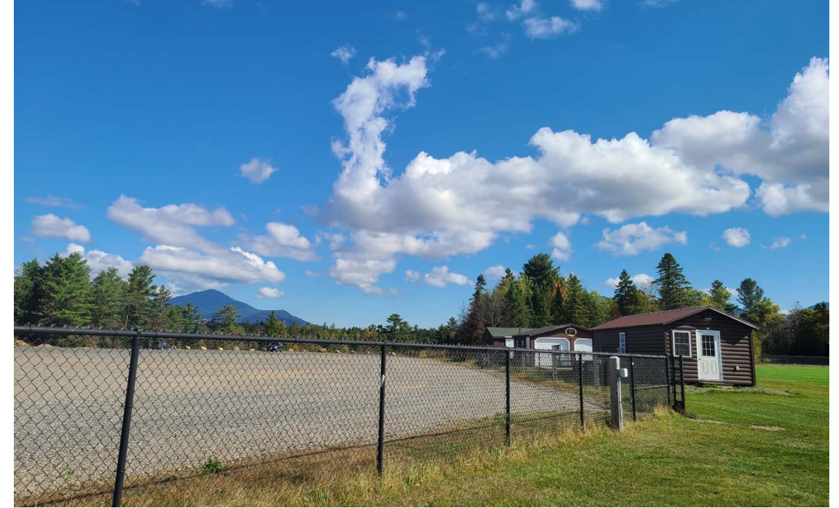
Buildings and Storage at Athletic Fields
