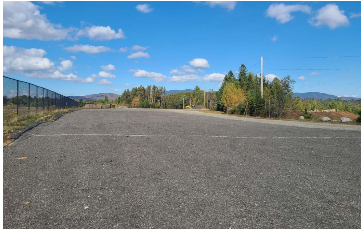
Overflow Parking Area (looking North-West)
