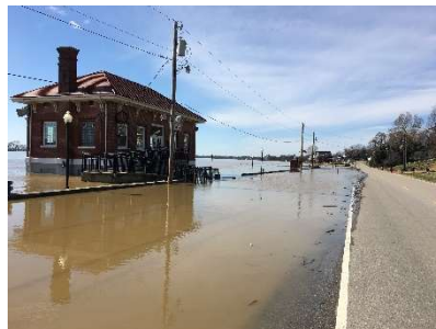
Figure 4 Trail in front of Old Lock and Dam Control Building No. 47 Under Water 2018
