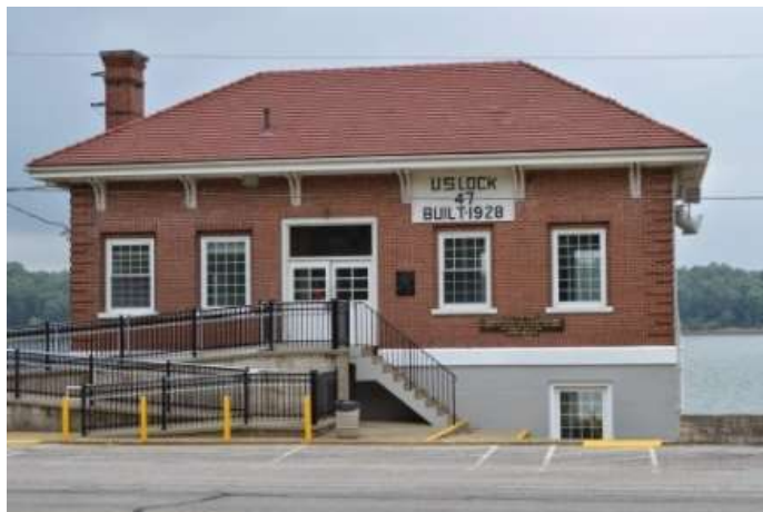
Figure 34 – Old Lock and Dam Control Building No. 47
