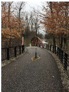
Figure 3 Historic Bridge No. 264 Under Water 2018
