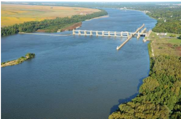
Figure 8: Newburgh Locks and Dam. Lrl.usace.army.mil
