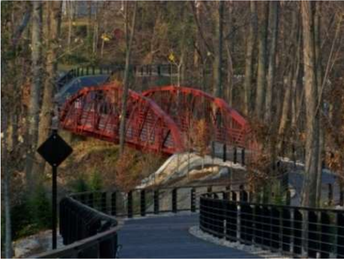
Figure 10: Warrick County Historic Bridge No. 264 Newburgh Museum Photo
