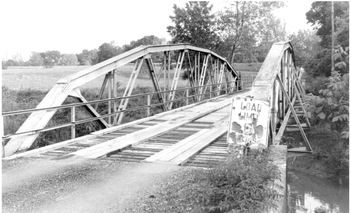
Figure 11: Warrick County Historic Bridge No. 264. Previous Location
