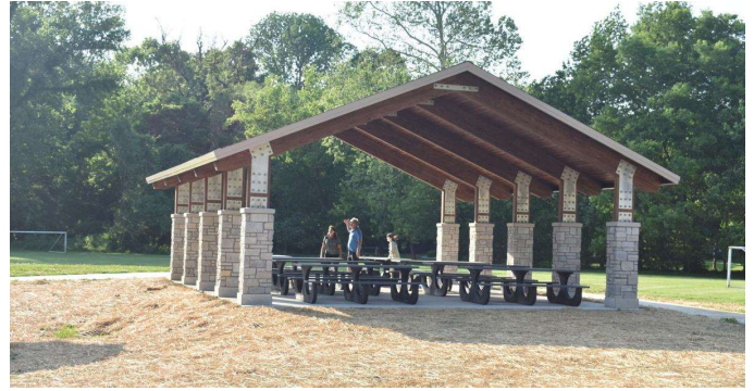
Figure 32 – Kiwanis Club of Historic Newburgh Picnic Shelter
