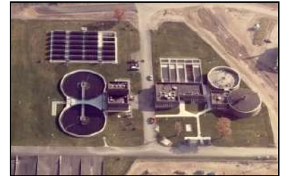
Waste Water Treatment Plant
