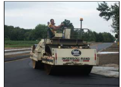
Repaving of Street
