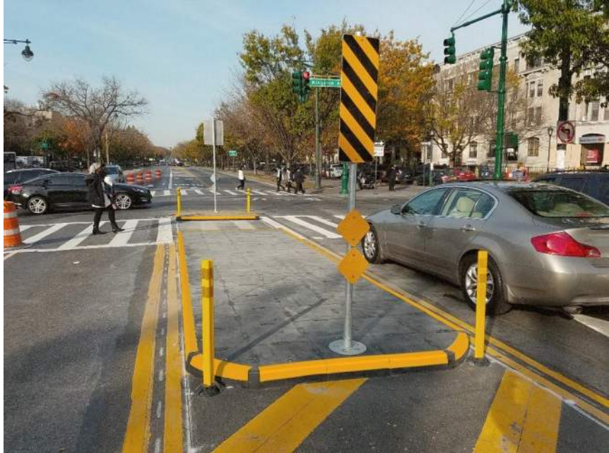
Figure 35: Temporary Median Installation
