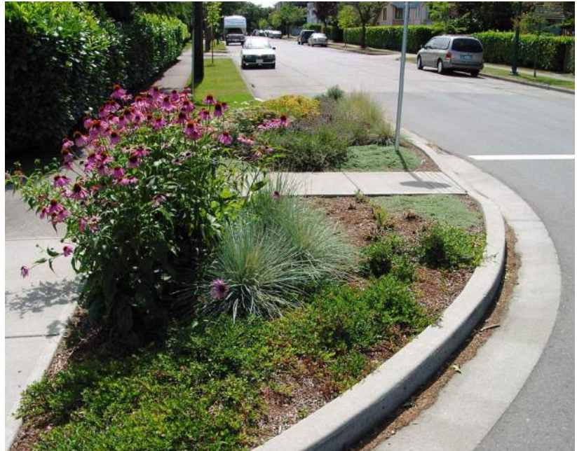
Figure 17: Curb Extension at Intersection
