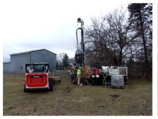
Rotosonic drilling at MW-201 (4/11/2022).
