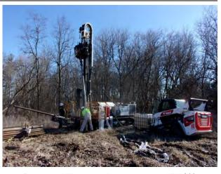
Rotosonic drilling and soil core retrieval at MW-200 (4/12/2022).
