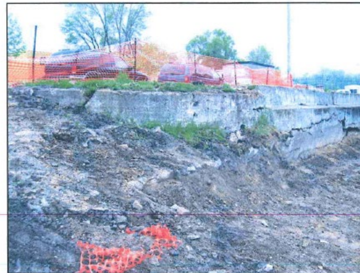
PHOTO NO. 12: East Wall - Eastern End
