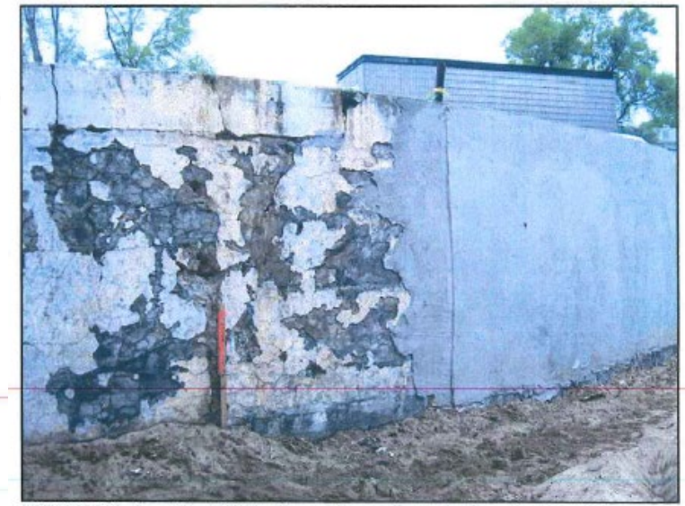
PHOTO NO. 4: West Wall - Transition to Concrete Repairs
