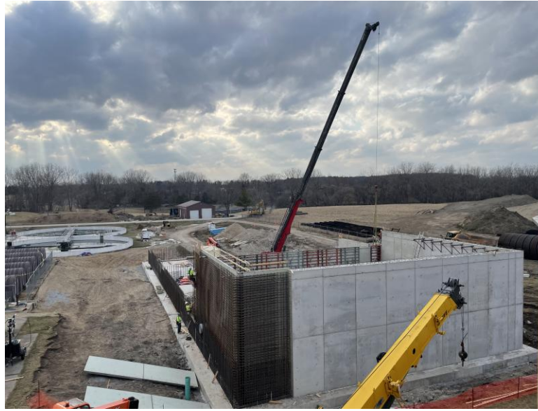
AGS Wall Construction
