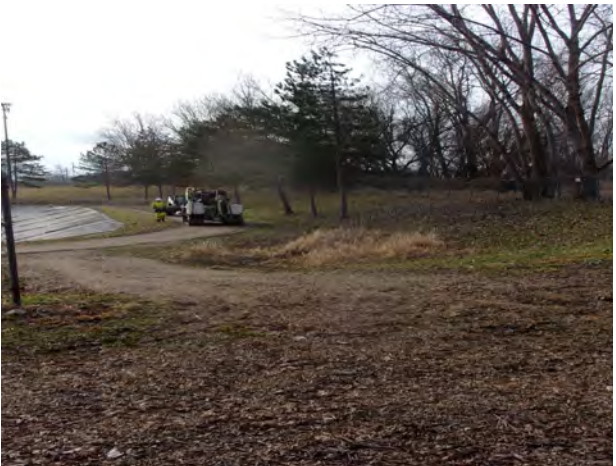
Tracking to SB-21 boring location (4/13/2022)
