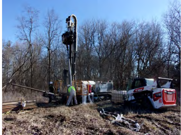
Rotosonic drilling and soil core retrieval at MW-200 (4/12/2022).
