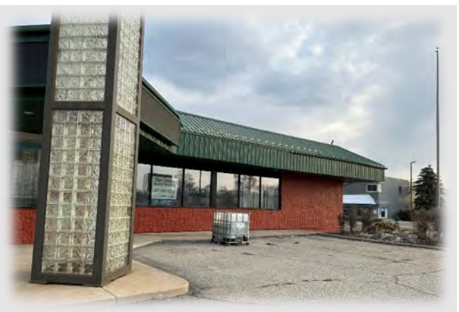
317 N Mission Street viewed from the parking lot, looking north (March 2023).
