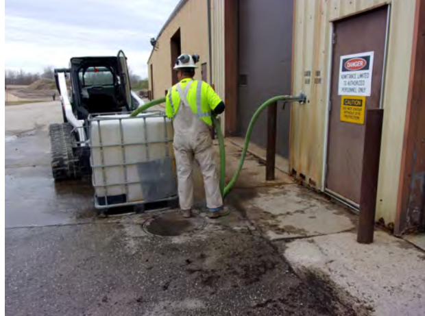
Rotosonic drilling potable water supply at Mt. Pleasant vehicle maintenance garage (4/11/2022).
