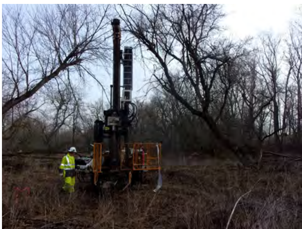
Drilling at SB-21 (4/13/2022).
