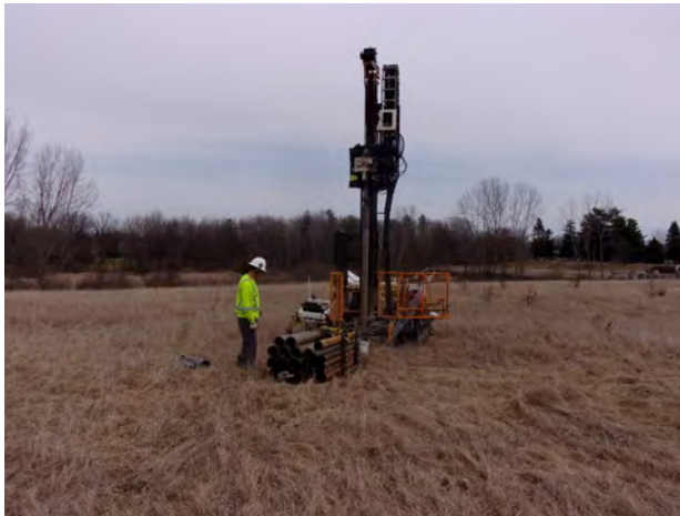
Setting up the rotasonic drill rig at the SB-19 boring location (4/12/2022).
