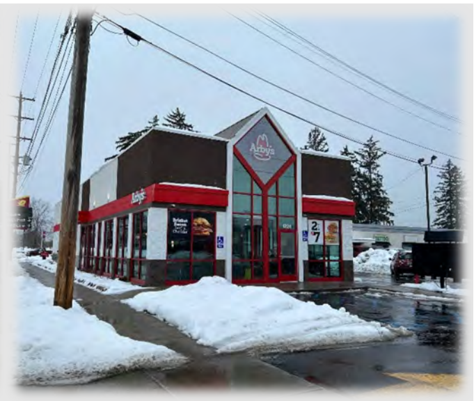
1224 S Mission Street after renovations, viewed from E Preston Street looking northwest (January 2024)
