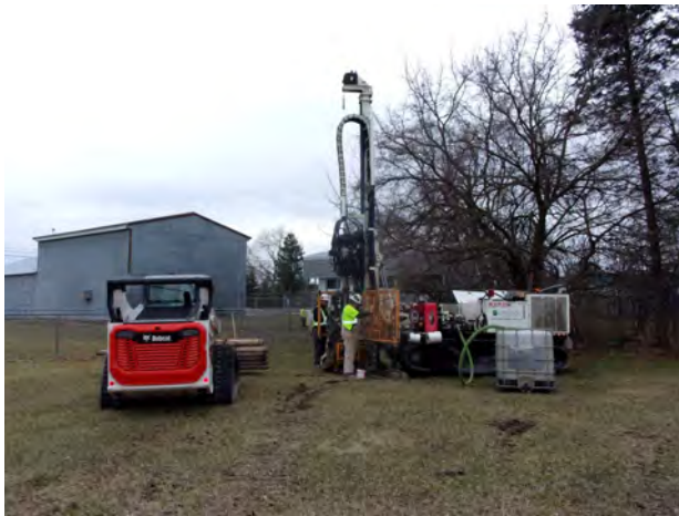
Rotosonic drilling at MW-201 (4/11/2022).
