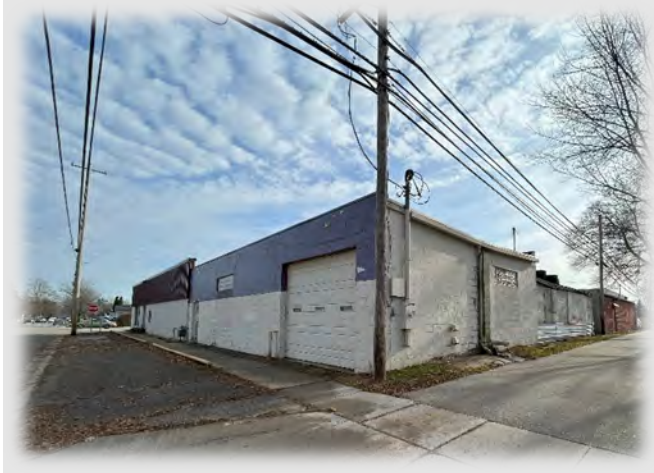
317 N Mission Street viewed from E Lincoln Street looking southwest (December 2023).
