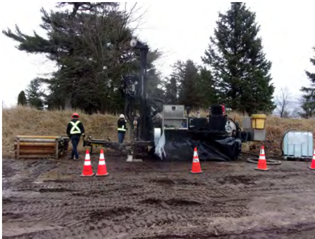
Rotasonic drilling and soil sampling at MW-300 (4/4/2023).
