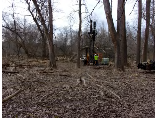
Drilling at MW-202 location (4/12/2022).
