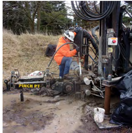
Tremie grouting annular space at MW-300 (4/5/2023).
