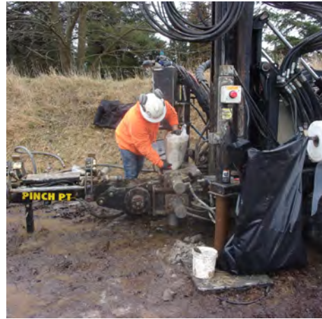
Installing filter sand in annular space at MW-300 (4/5/2023).
