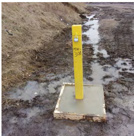
Monitoring well MW-300 looking south (4/5/2023).
