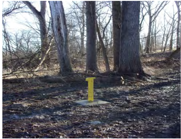
Monitoring well MW-202 (4/14/2022).
