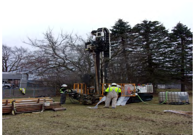
Drilling and retrieving soil core at MW-201 (4/11/2022).
