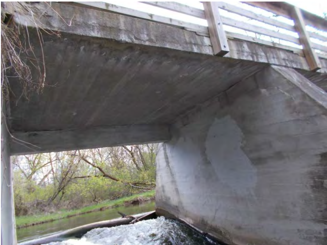
View of east span from northeast bank area
