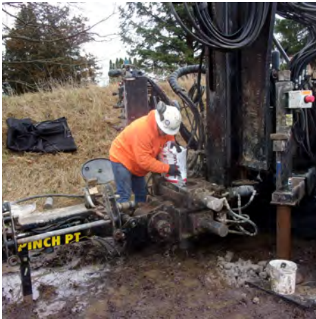
Installing bentonite chip seal in annular space at MW-300 (4/5/2023).
