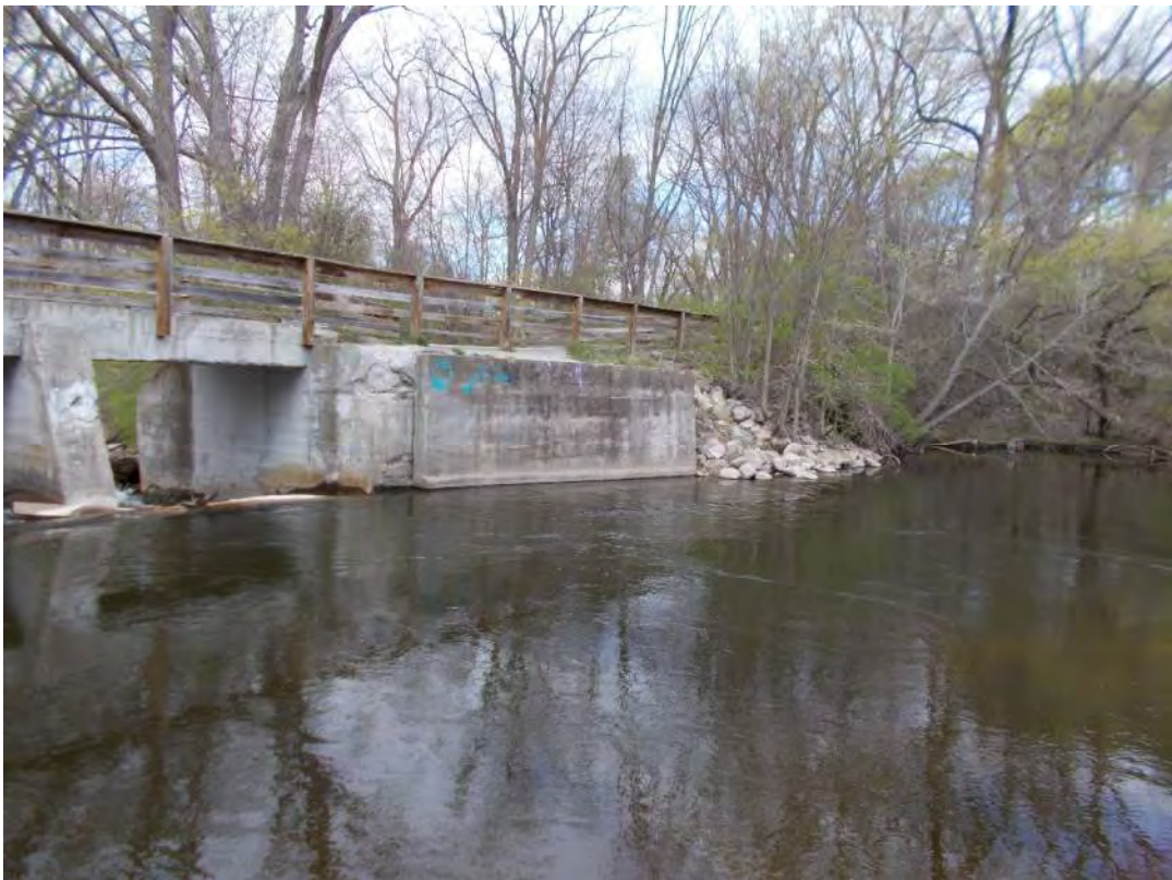
View of southeast wingwall looking northeast
