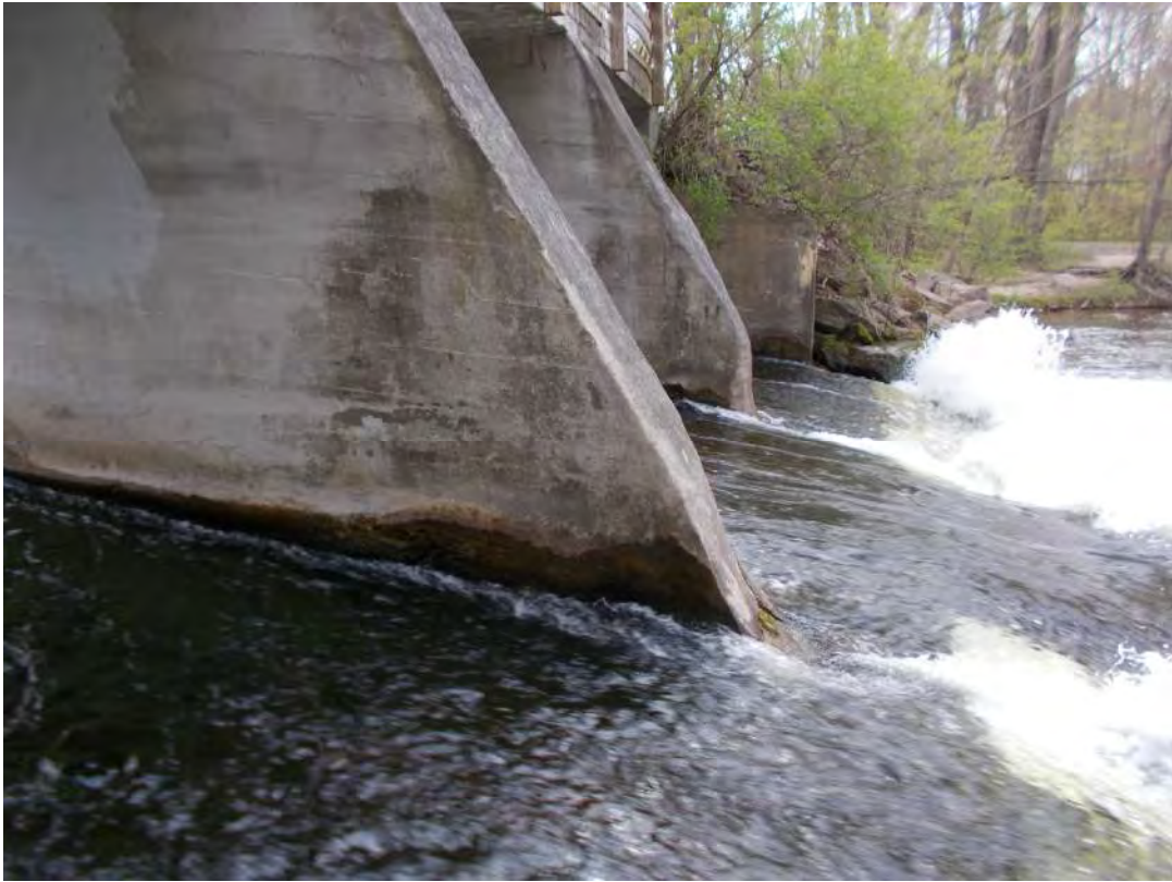
View of spillway area looking west
