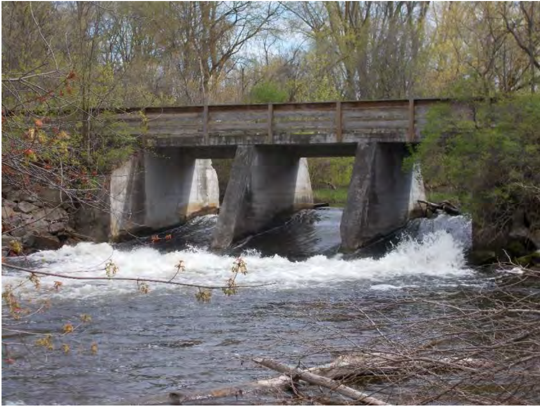
Elevation view of structure looking south
