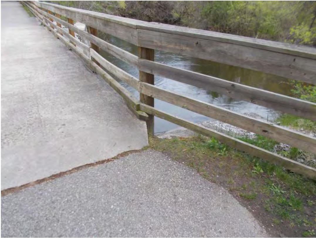
View of southwest railing transition area
