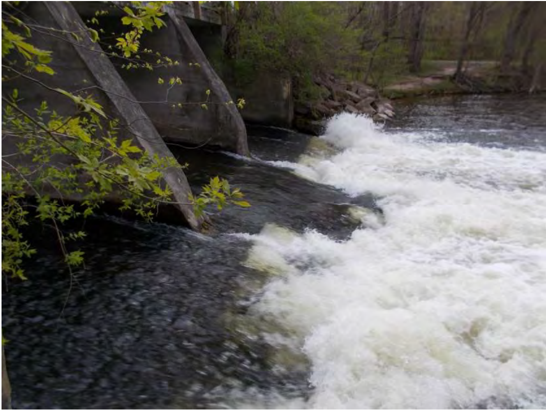
View of downstream spillway area looking west
