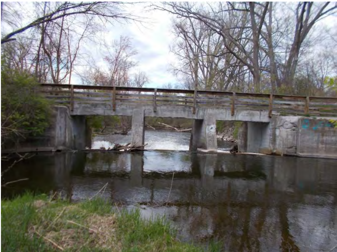
Elevation view of structure looking north
