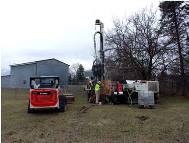
Rotosonic drilling at MW-201 (4/11/2022).
