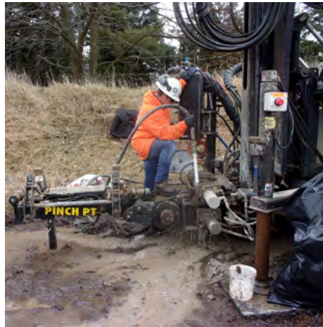
Tremie grouting annular space at MW-300 (4/5/2023).
