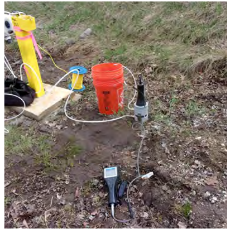
Purging Deep Monitoring Well MW-300 (4/20/2023).
