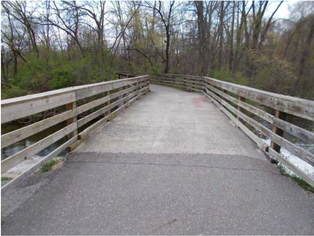
View of structure from east approach
