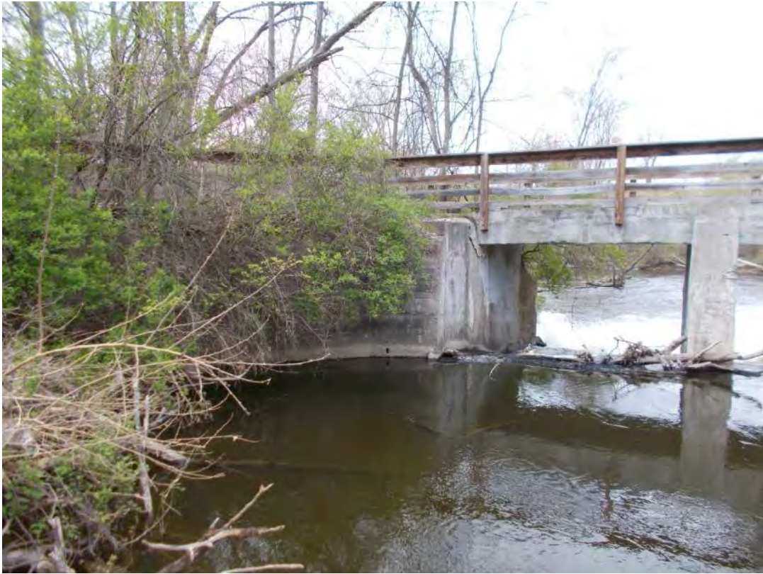
View of southwest wingwall area looking north
