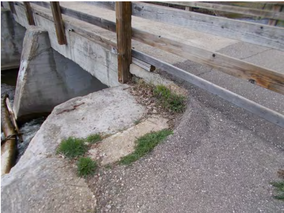
Asphalt curbing/spillway area in southeast
