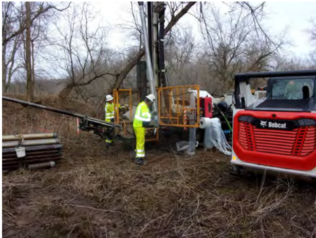
Retrieving soil core at boring SB-21 (4/13/2022).
