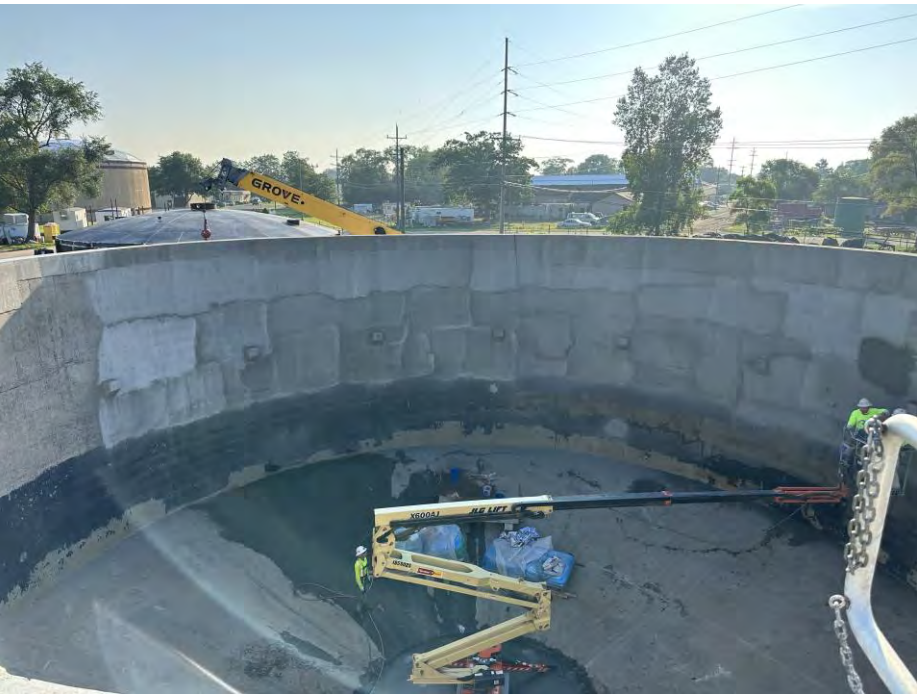
Rehabilitation of the Primary Digester
