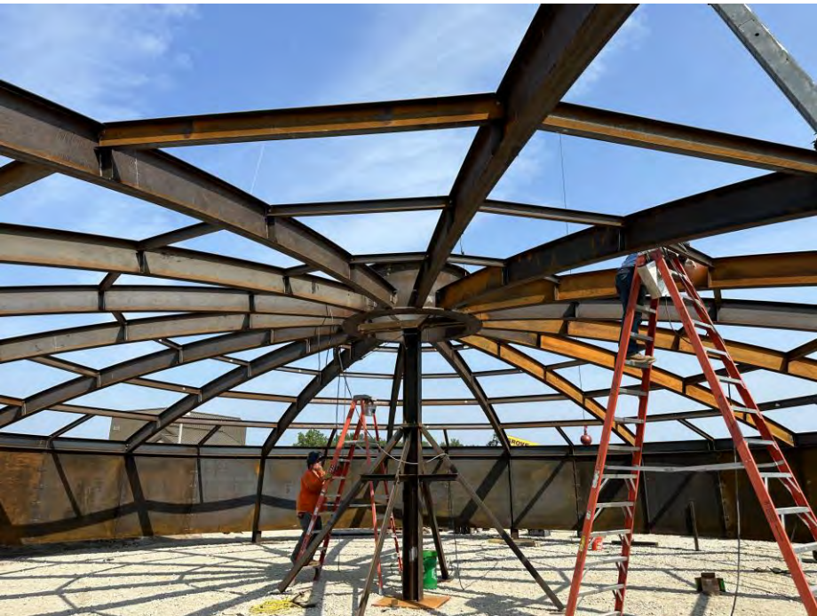
Digester Lid Construction Inside
