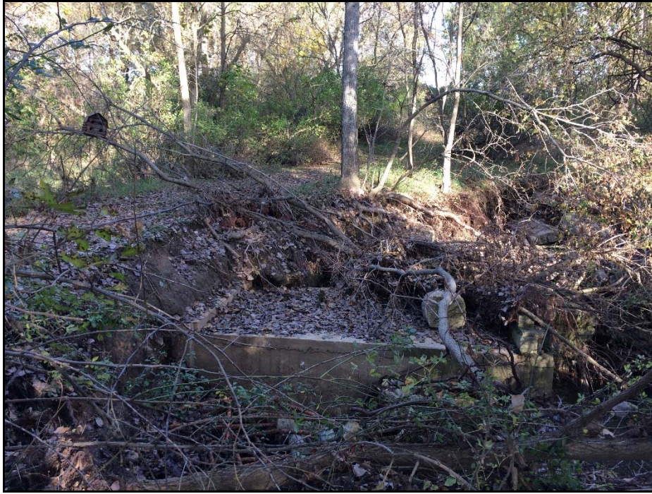
Photograph 11 – Erosion on downstream slope adjacent to principal spillway, viewed from right
