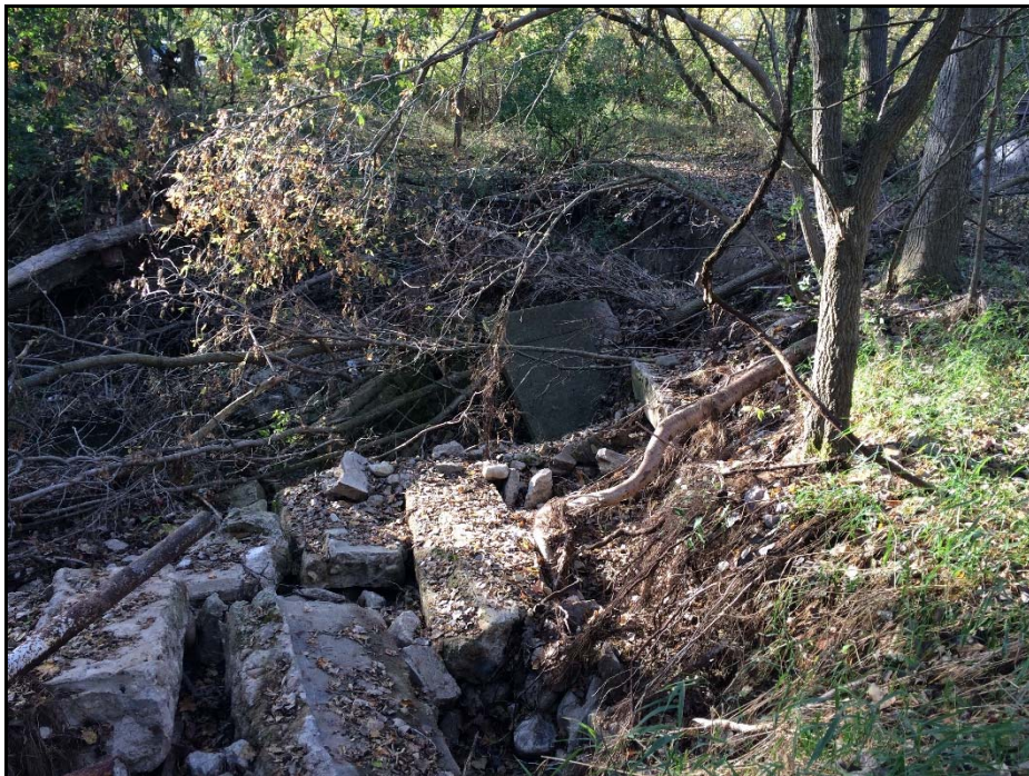
Photograph 10 – Erosion on downstream slope adjacent to principal spillway
