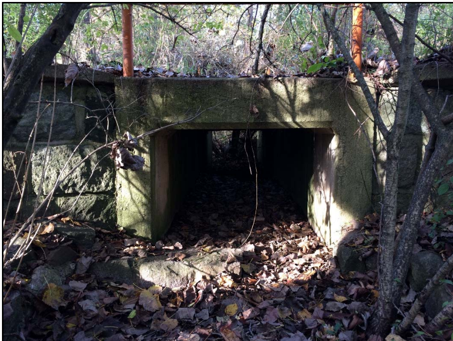
Photograph 16 – Outlet end of auxiliary spillway
