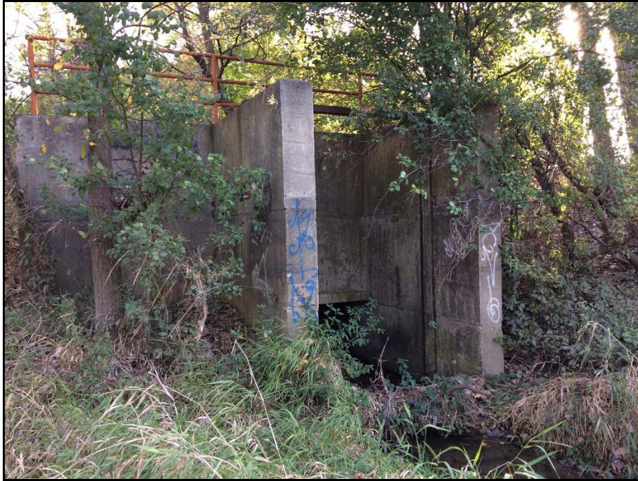
Photograph 3 – Principal spillway entrance
