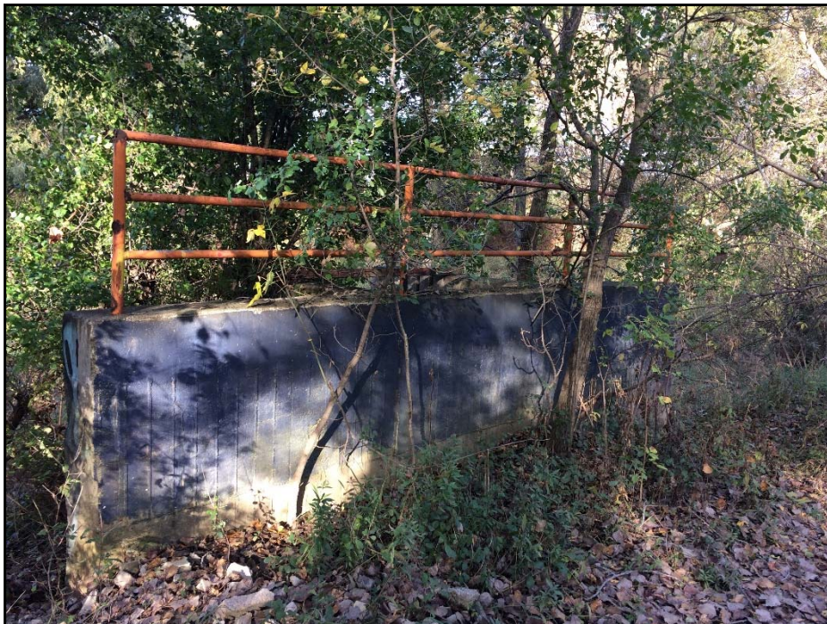
Photograph 6 – Downstream face of principal spillway headwall
