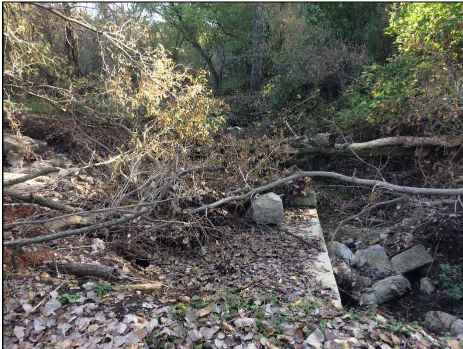
Photograph 12 – Erosion on downstream slope adjacent to principal spillway, viewed from embankment crest, looking downstream
