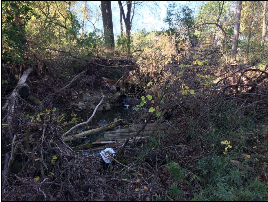
Photograph 9 – Erosion on downstream slope adjacent to principal spillway
