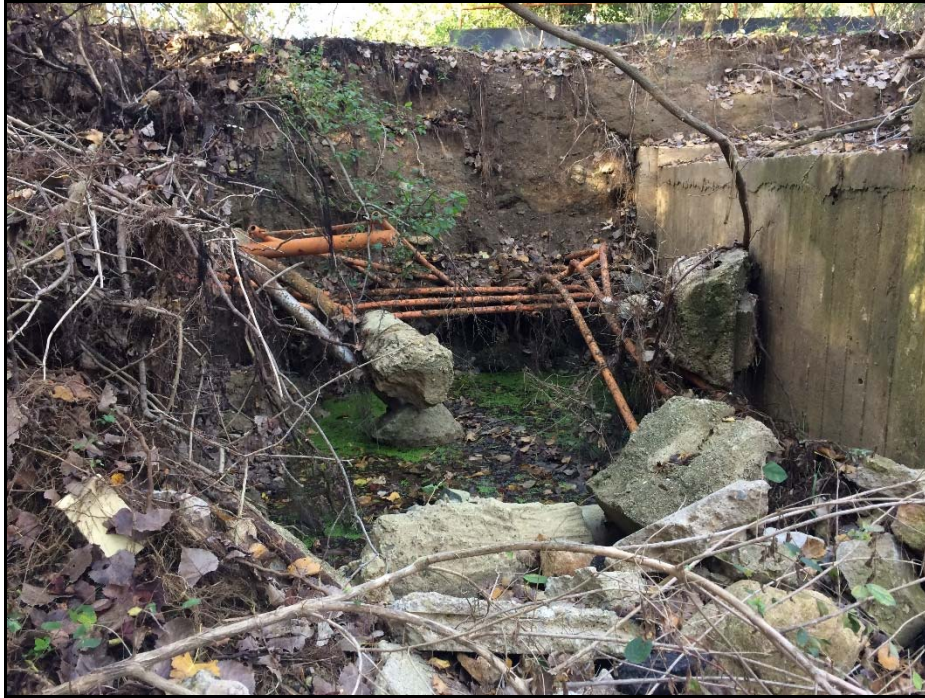
Photograph 13 – Debris on downstream slope
