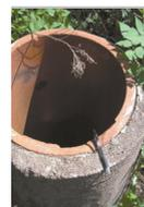
Dug wells typically appear as a ring anywhere from 1 foot or several feet in diameter, made of concrete, tile, bricks, or rocks
