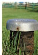
Pipes 1 to 8 inches wide above, at, or below the surface may indicate a well (sewer lines or septic systems may also have similar pipes, investigate further if unsure)
