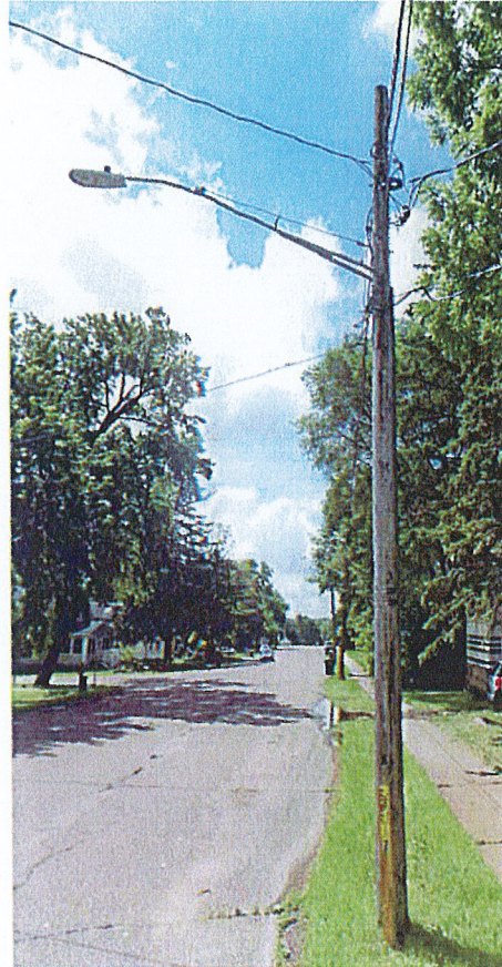
Picture 2: Intersection Street Light on Wood Overhead Electric Distribution Pole
