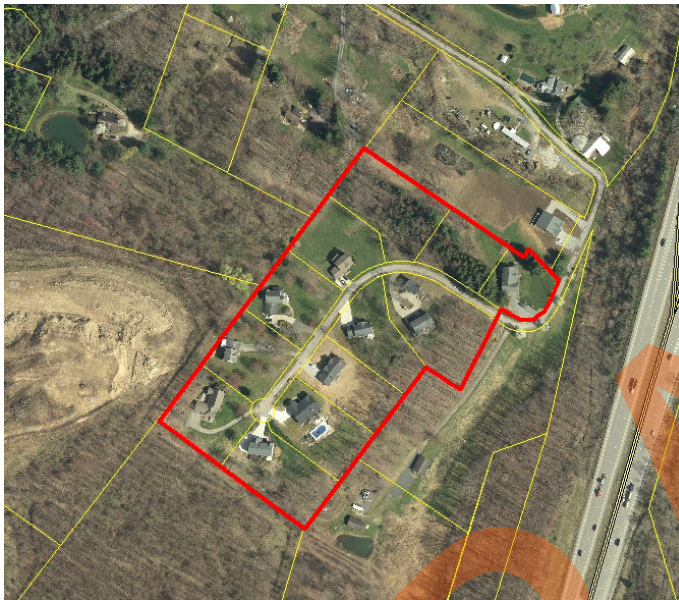
The 12 parcel development at right shows a typical example of an unphased Major Subdivision
