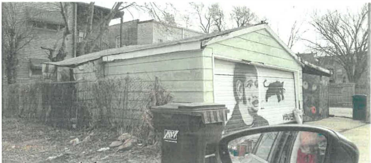
Rear garage showing severe dilapidation and breach of north facing wall, making it subject to the elements, including water intrusion.
