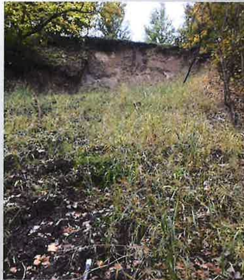
Large Scarping of Side slope
