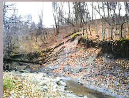
Large Scarping of Side slopes
