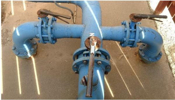
Cast-iron piping w/ lever valves
