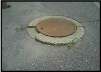
Traffic Signal Handhole
