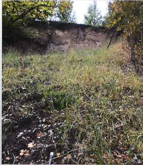
Large Scarping of Side slope
