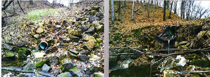
Correct Outlet Piping
