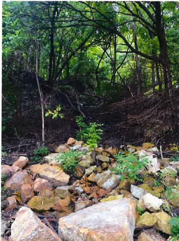
Rip-rap installed around inlet and upstream from inlet
