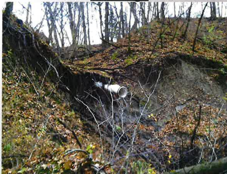
Outlet That Needs Correction
