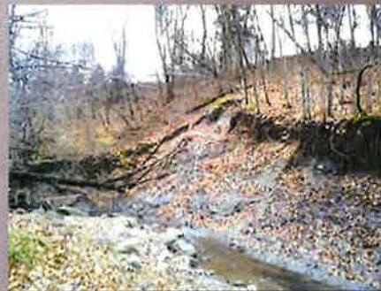
Large Scarping of Side slopes
