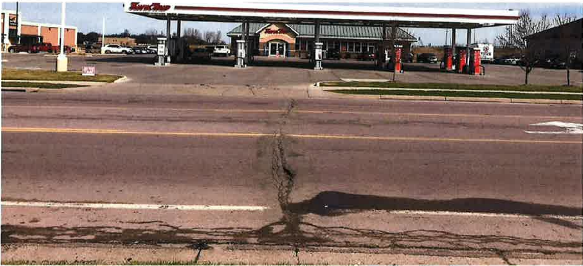
Another view of deteriorating roadway and driveway pavement between Lor Ray Drive and Roe Crest Drive, showing potential drainage issues along the shoulder/curb line.
