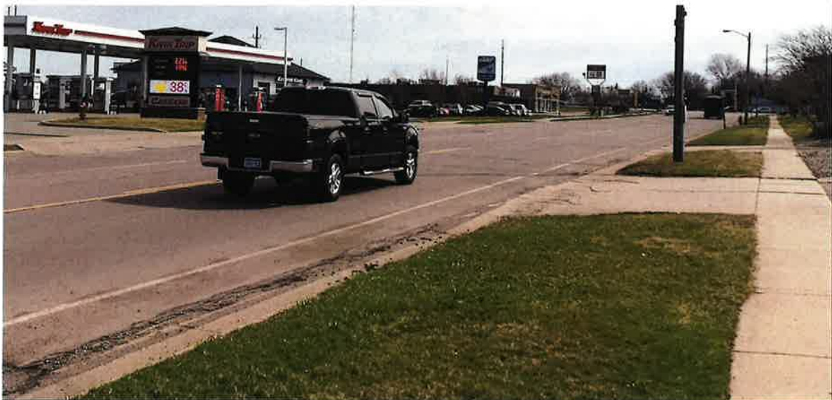
View of deteriorating pavement and driveways, many nearby accesses, non-compliant pedestrian facilities and existing lighting looking north east from east of Lor Ray Drive.
