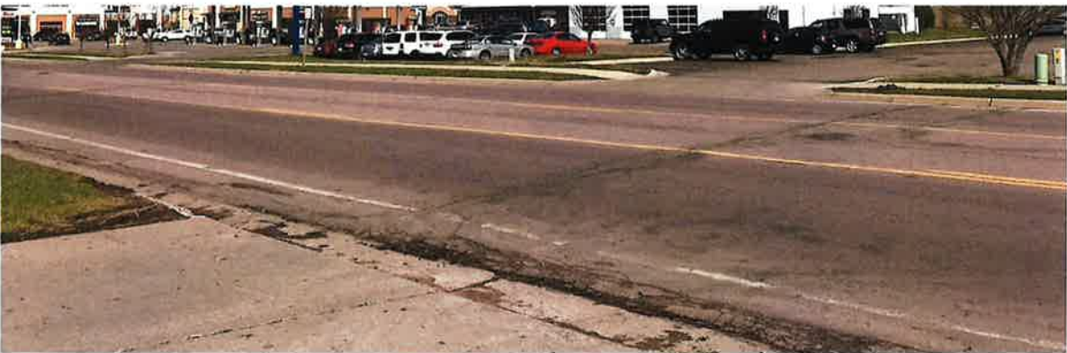
View of closely spaced and offset accesses with more areas of deteriorating pavement just west of Lor Ray Drive.
