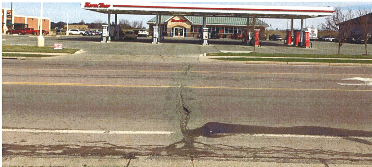
Photo 3 - Another view of deteriorating roadway and driveway pavement between Lor Ray Drive and Roe Crest Drive, showing potential drainage issues along the shoulder/curb line.
