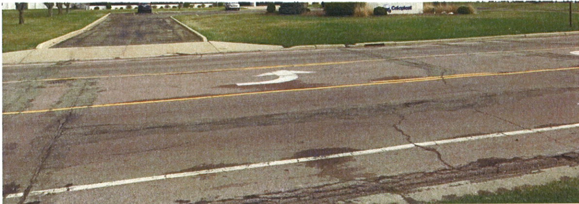
Photo 1 - View of deteriorating pavement on Commerce Drive west of Tower Drive.
