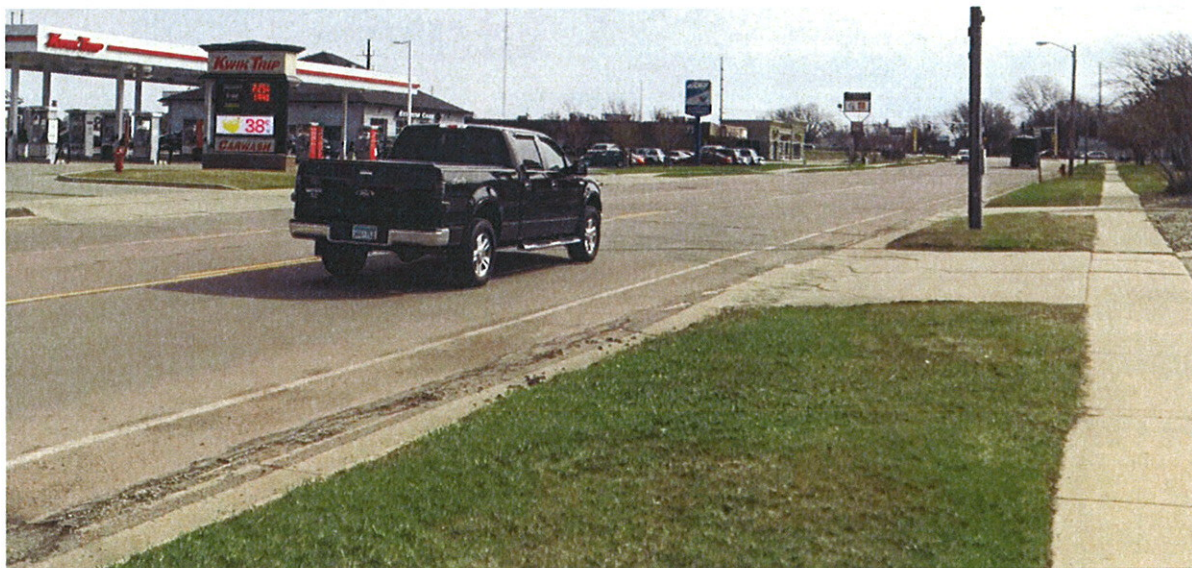
Photo 2 - View of deteriorating pavement and driveways, many nearby accesses, non-compliant pedestrian facilities and existing lighting looking north east from east of Lor Ray Drive.
