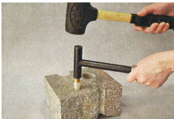
Figure 2. Installing the Vapor Pin™.
