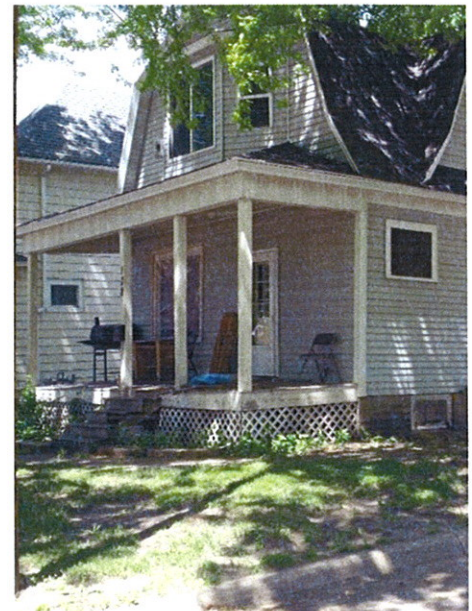
Figure 11. Renter-Occupied Home in Lower North Mankato. The stairs leading to the front entryway are broken and do not have a railing, paint is in poor condition, front window to home is in disrepair, and lawn is in poor condition among other things.
