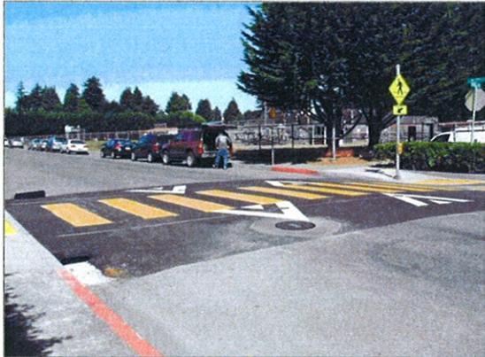
**Raised Crossing.** A raised pedestrian crossing is essentially a speed table or a speed hump with a flat portion the width of a crosswalk (typically 10' to 15' wide). Gently sloping ramps about 6' wide are placed on either side of the raised crossing. The raised crossing is generally at the same height as the sidewalk, while speed tables or bumps are typically between 3 to 6 inches.
