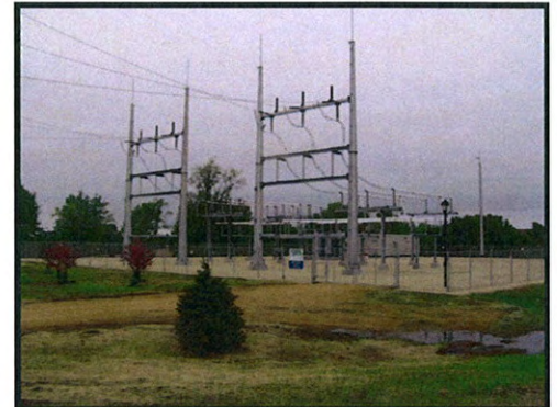
Figure 1 Typical 115 kV distribution substation
