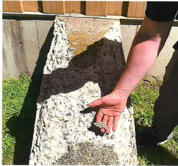
Deterioration at Concrete Buttresses
