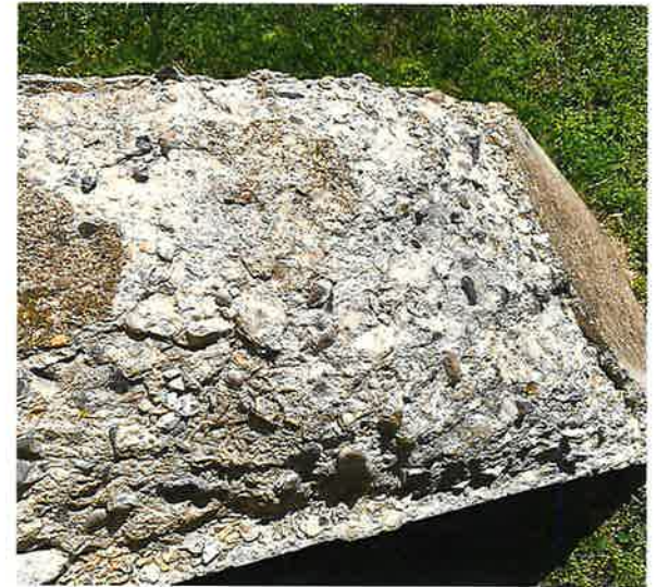
Deterioration at Concrete Buttresses
