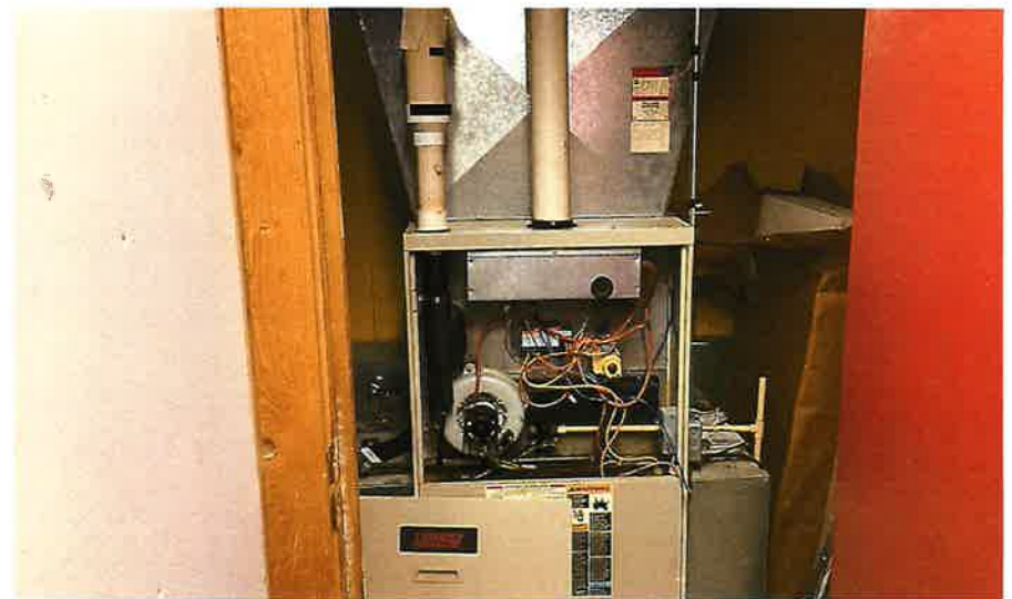
Condensing Furnace
