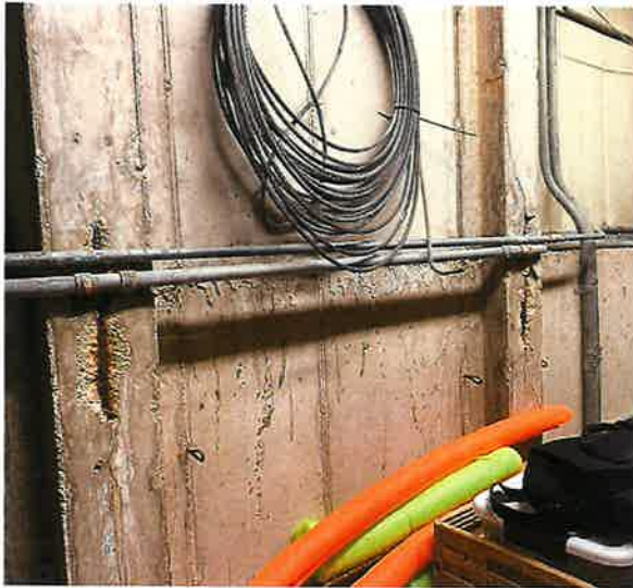
Deterioration of Concrete Below Bleachers
