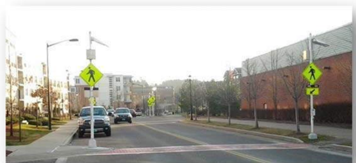
Figure 18. Ground-Mounted Rectangular Rapid Flashing Beacon
