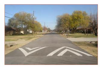
**Figure 18: Temporary Speed Lumps**
