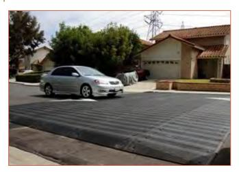
Figure 19: Temporary Speed Table
