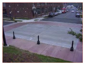
RAISED INTERSECTIONS are like speed tables that cover an entire intersection. Ramps are present on all approaches. The flat-top area is usually a textured material. Raised intersections usually rise to sidewalk level or slightly below to provide an edge for the visually impaired. If there is a concern about loss of on-street parking, raised intersections are a more acceptable traffic calming measure.
