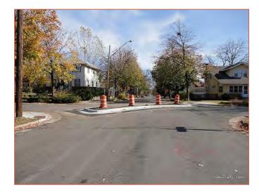
Figure 12: Diagonal Diverter
