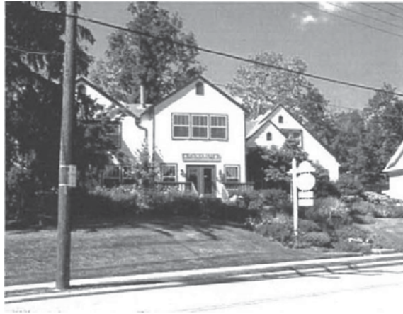
Figure 21: Example of a larger building along Laurel Avenue with appropriate articulation. A regular fenestration pattern which reflects the patterns evident in the existing residential structures can also add horizontal articulation to a building
