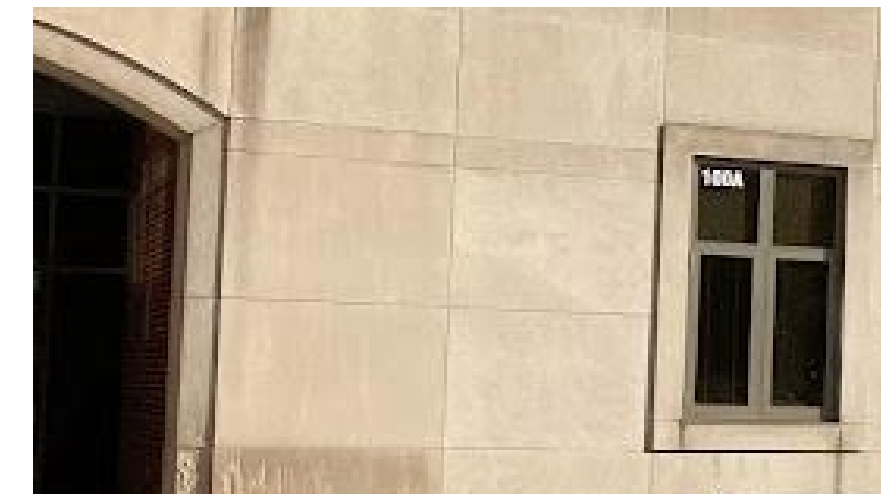
Stone Veneer Panels and Framing
