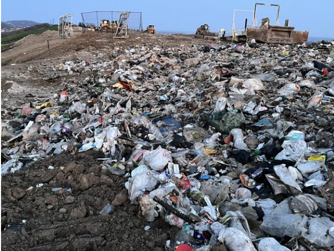
Photo 9: Uncompact/exposed waste adjacent to the tipper.
