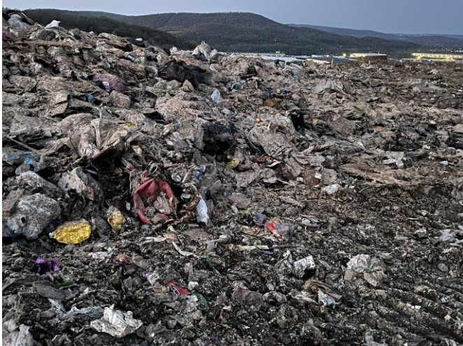
Photo 1: Uncompacted waste with minimal foam ADC at the active face.
