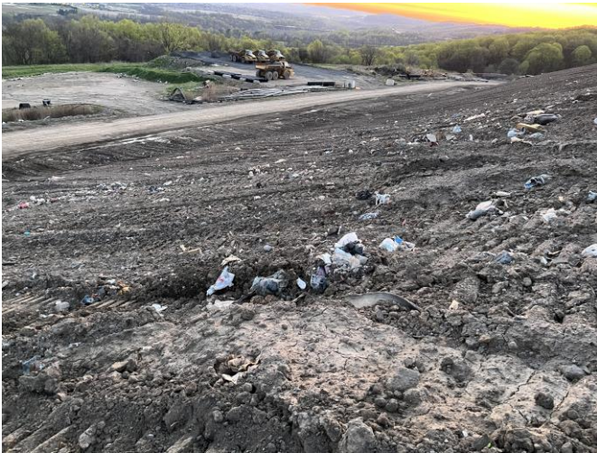
Photo 10: Exposed waste on intermediate cover on the north slope.
