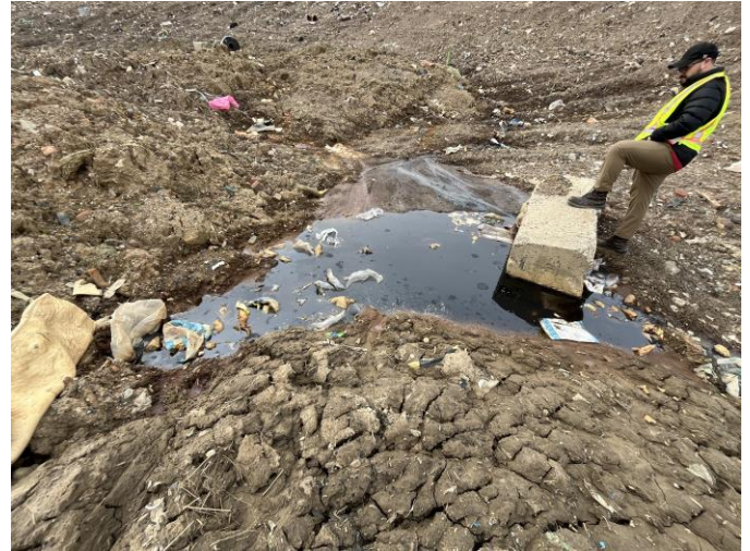
Photo 11: Leachate seep adjacent to access road north of disposal area.
