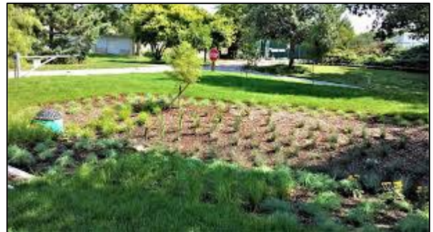
Dry detention pond with planted bottom
