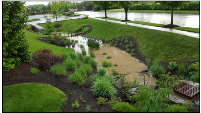
Wet pond in a commercial development acting as a first point of treatment. Note the inclusion of several species of trees and shrubs.
