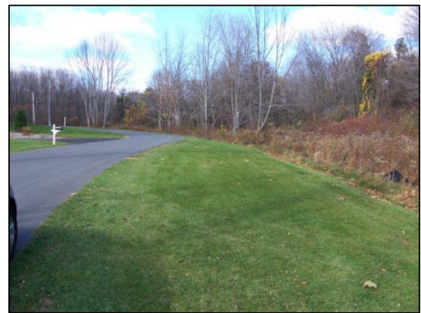
Vegetated filter strip in a residential setting
