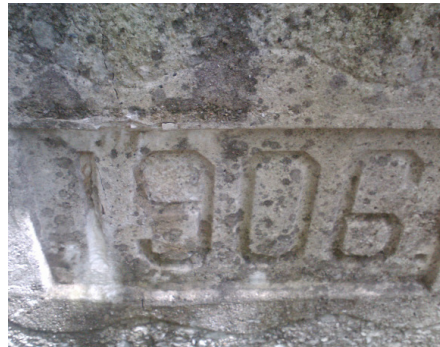
Outside of Dellwood Park bridge
