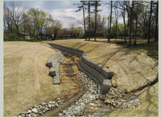
Rose Tree Outfall Project
