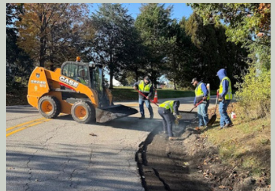
Asphalting along Savage Road
