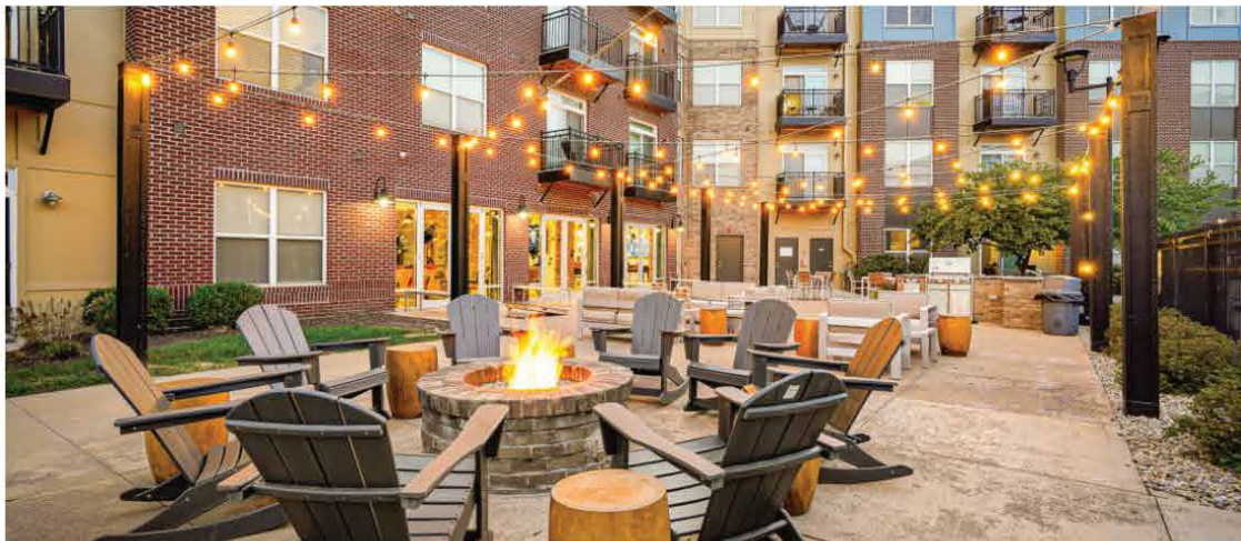
Three- and four-story masonry buildings with a combination of gable end and parapet roofs, repetitive window treatments, and outdoor gathering spaces.
