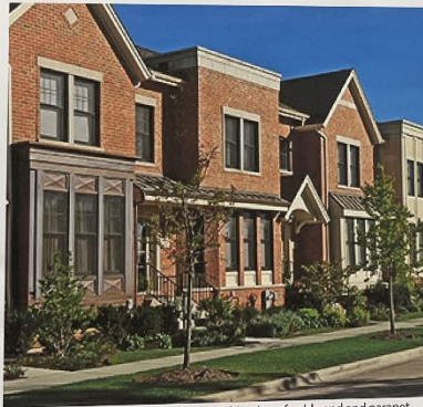
Two-story masonry buildings with a combination of gable end and parapet roofs, pronounced porches, window bays and landscaped front yards and parkways.
