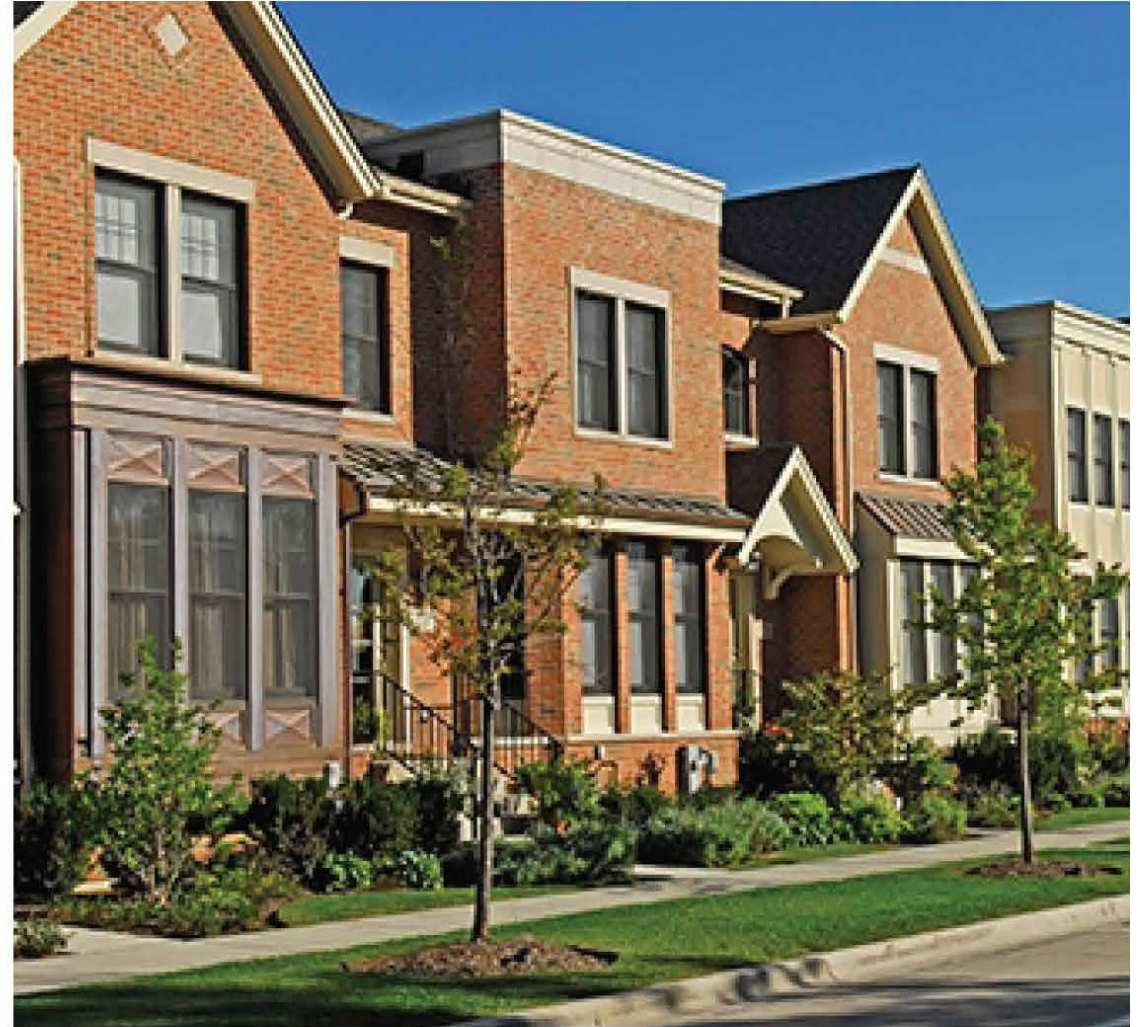
Two-story masonry buildings with a combination of gable end and parapet roofs, pronounced porches, window bays and landscaped front yards and parkways.
