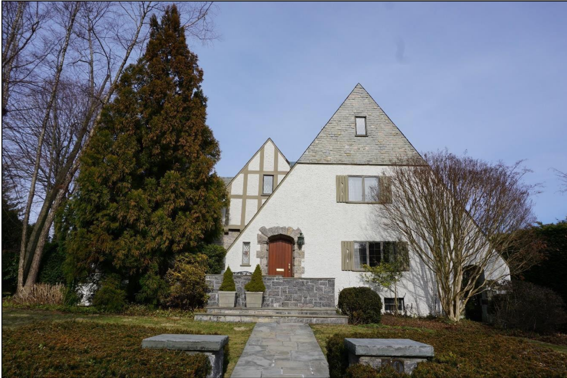
Fig.16: Unnamed house, 10 Elm Ave., ca. 1927.
