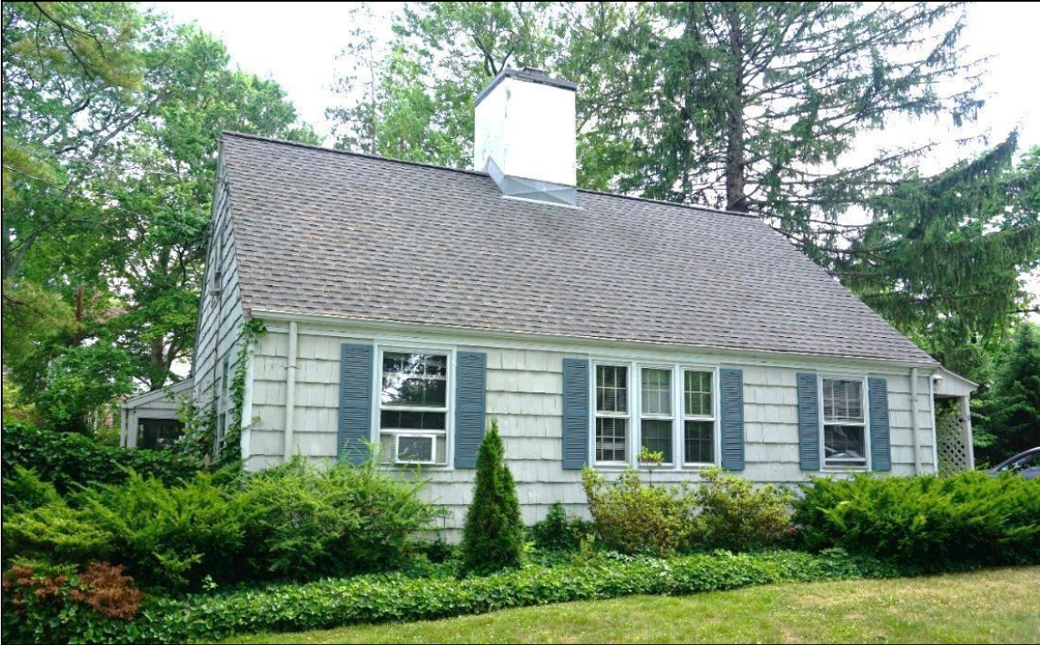
Fig.21: Unnamed house, 9 Cedar Ave., ca. 1920.
