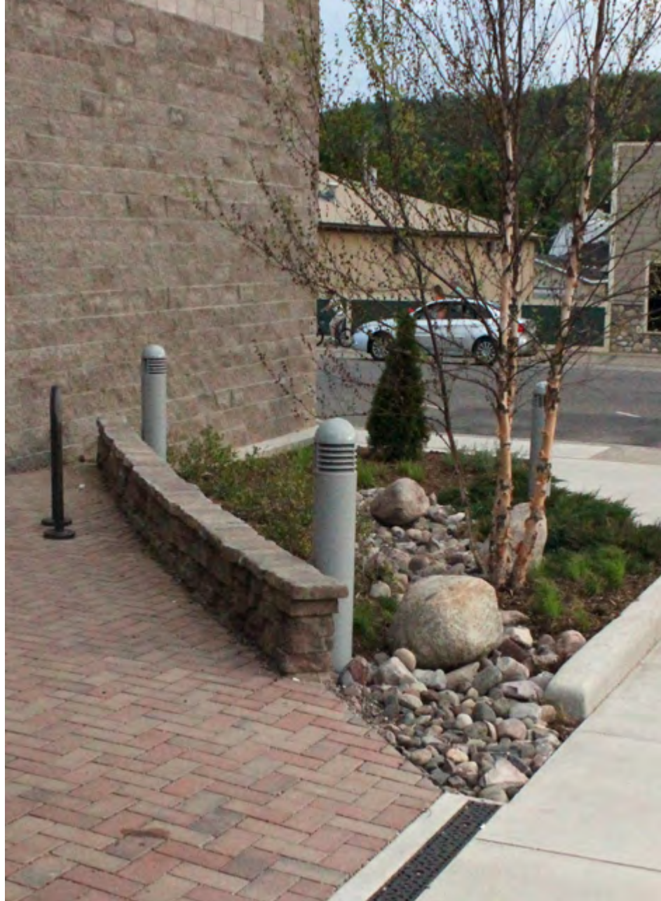
FIGURE 9.4 - BUS STOP IN MUNISING CONVERTED TO UTILIZE POROUS PAVEMENT WITH A RAIN GARDEN
