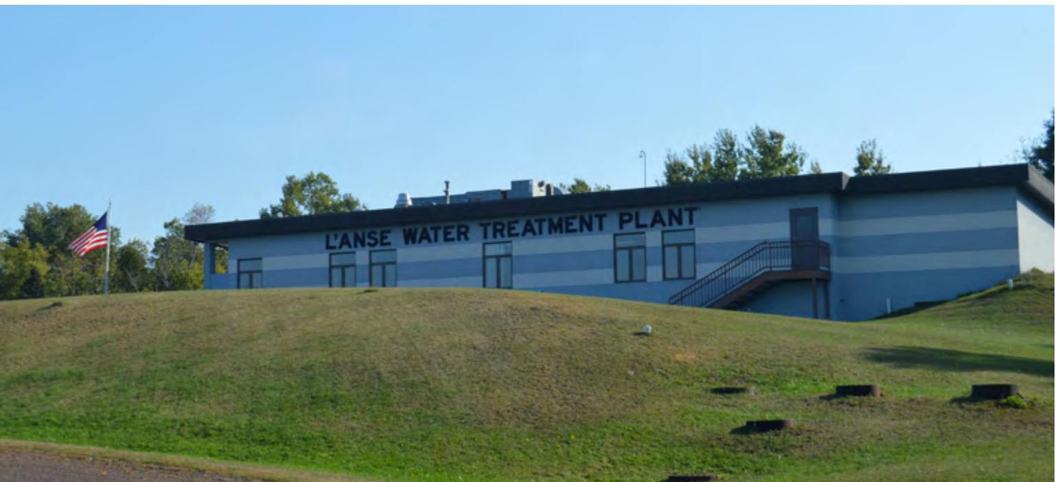
FIGURE 5.0 L'ANSE WATER TREATMENT PLANT
