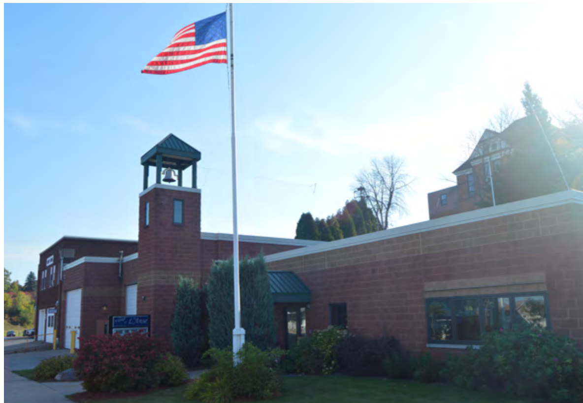
FIGURE 5.3 - VILLAGE HALL & FIRE STATION
