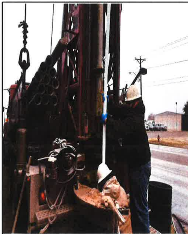
Typical well pipe installation process.
