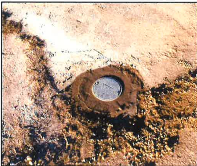
Typical well surface completion in asphalt/concreted area.
