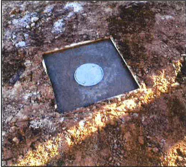
Typical well surface completion in dirt/grassy area.
