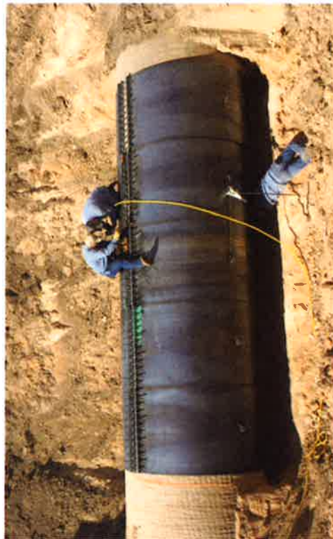
Full Pipe Clamp Repair
