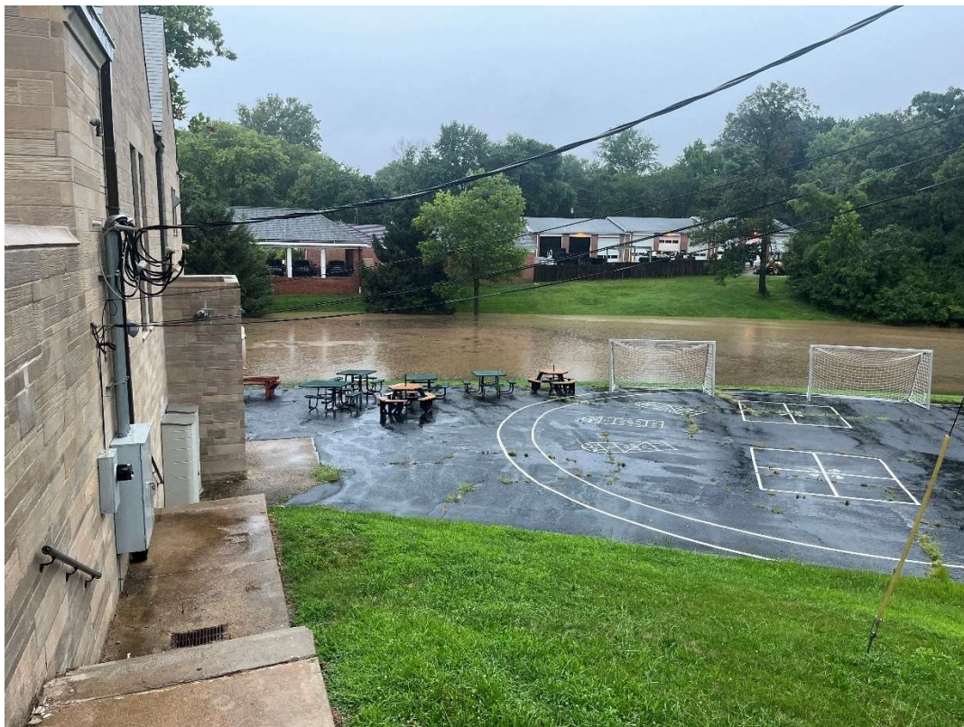
Figure 7: Photo taken of flooding between Church of the Annunziata Elementary School and City of Ladue Police Department. Photo taken on July 16, 2024. The proposed 1642-R24 Tributary 6 Storm Sewer Improvements Project will significantly reduce the potential for flooding of the Elementary School.
