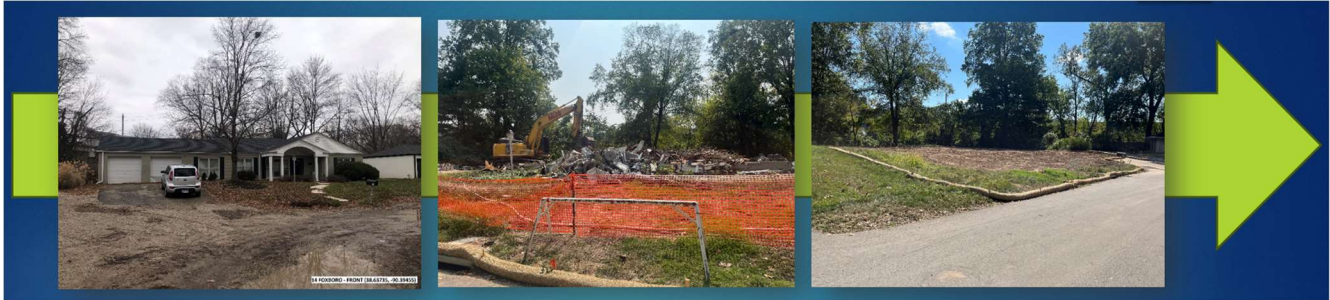
Figure 17: Before, during, and after the demolition of 14 Foxboro Road.
