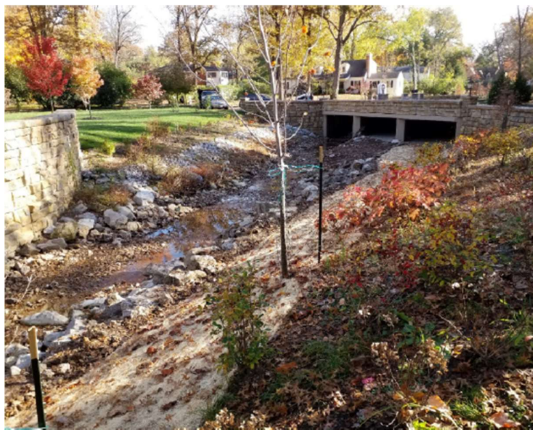
Figure 15: Completed view of Robin Hill Lane – McKnight Lane streambank stabilization improvements.
