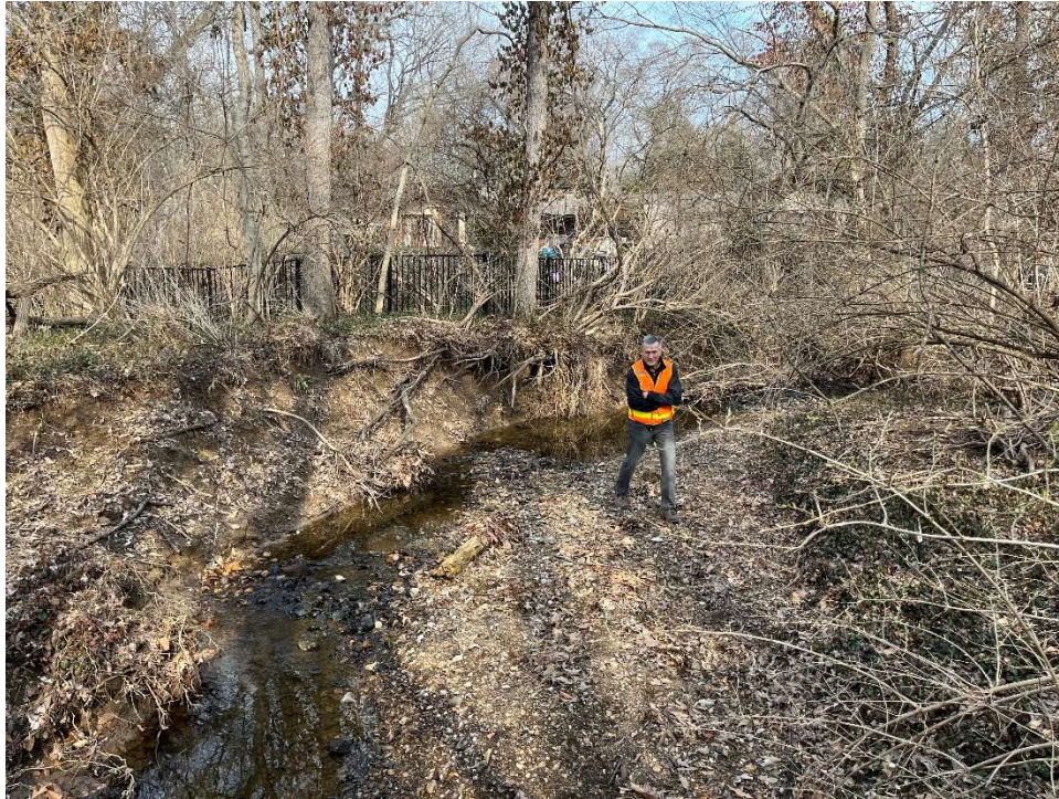
Figure 1: Public Works Stormwater Project Engineer Denny Welker performing a field investigation site visit in February 2024. The streambank behind Mr. Welker is an example of significant deterioration in need of streambank stabilization.
