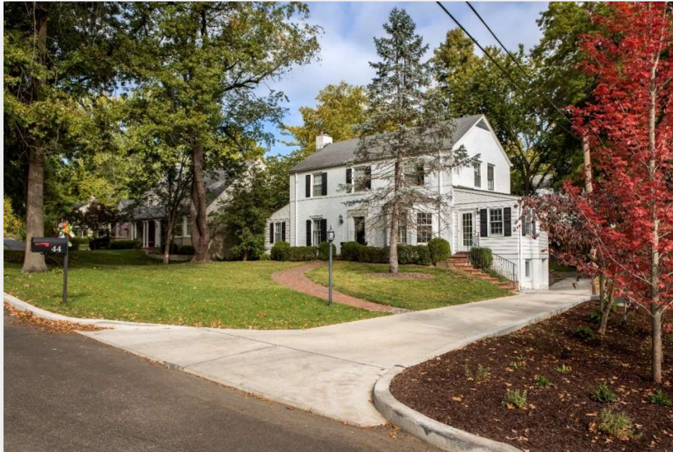
Figure 13: Photo taken after construction was completed at #44 Willow Hill Road. Prior to the project, this property had a history of severe structural flooding. Photo taken October 2022.
