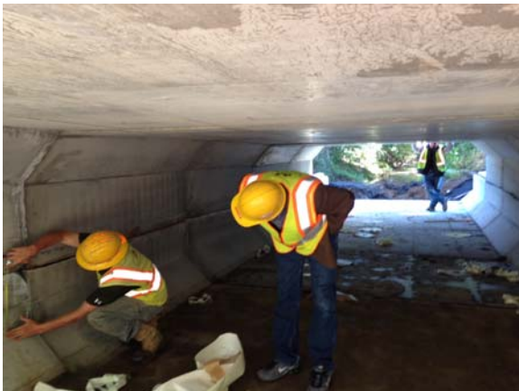
Installation of new Culvert
