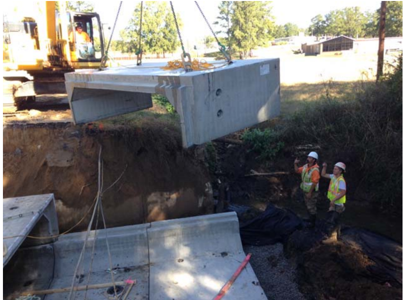
Emergency Culvert Replacement Construction
