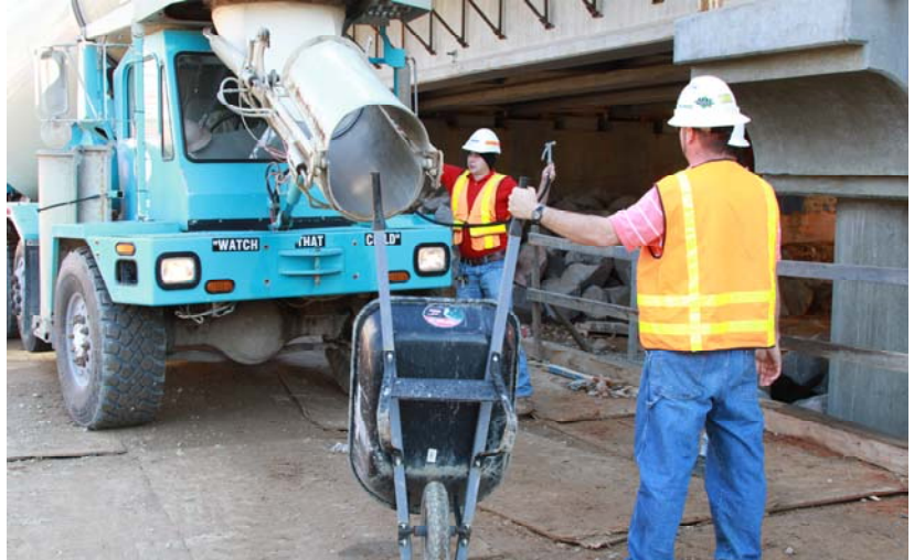
Concrete Testing for Broad River Road Bridge Project
