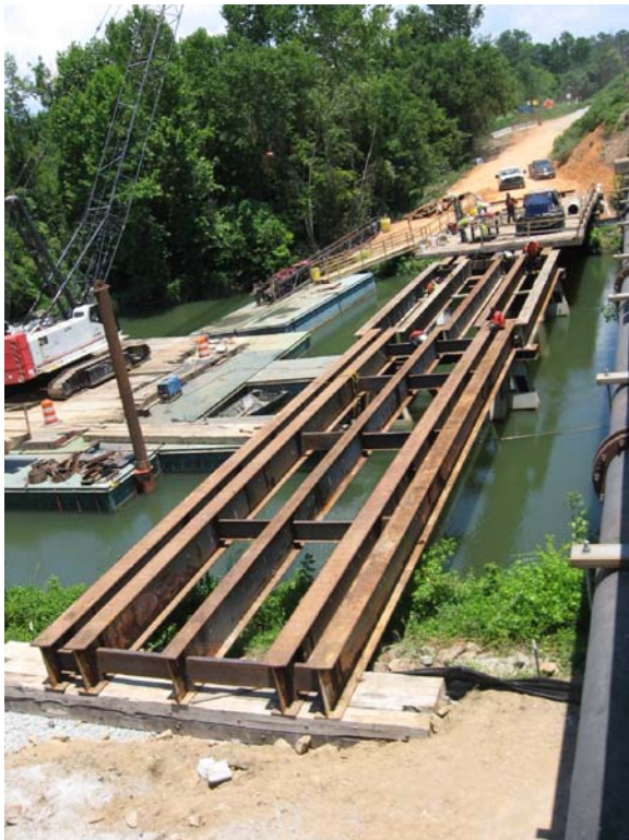
Temporary Bridge for Construction
