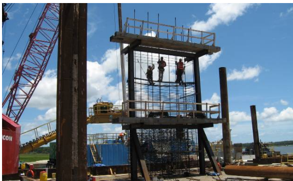
Building the Rebar Substructure
