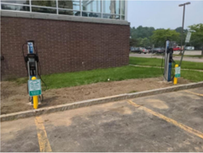
Siena College Charging Stations: Grass with Concrete Foundations.
