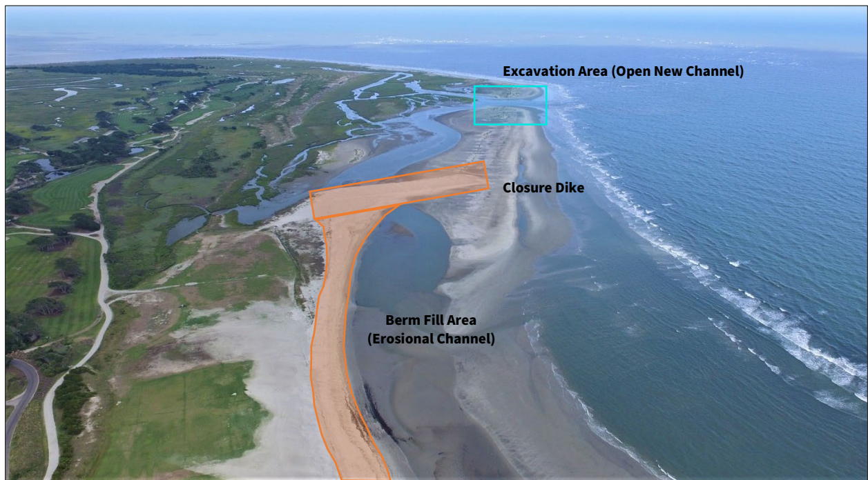
FIGURE 2.10. [UPPER] Excavation and fill areas used in the 2015 project. Approximately 100,000 cy of sand was transferred from the excavation area to the fill. [LOWER] Project area on 7 July 2015 after project completion showing closure dike in center of image and new flushing channel at upper right. Encroachment by the ‘erosional channel’ destroyed hundreds of feet of dunes, leaving no protection in front of the driving range.
