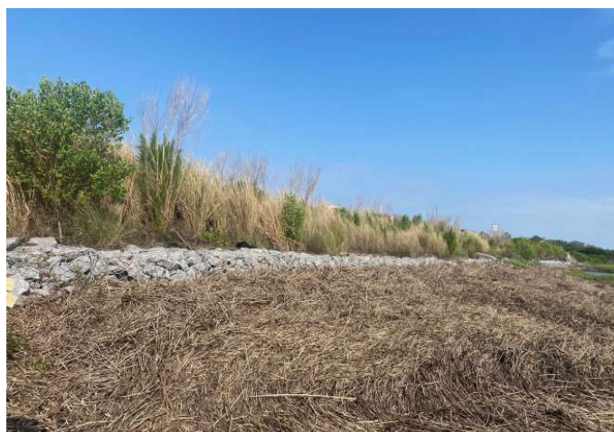
A revetment of vertical caged rock marks the transition from uplands to tidal area. Wack is trapped covering existing Spartina .
