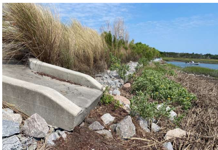
Stormwater outfall from Kiawah Island Parkway.
