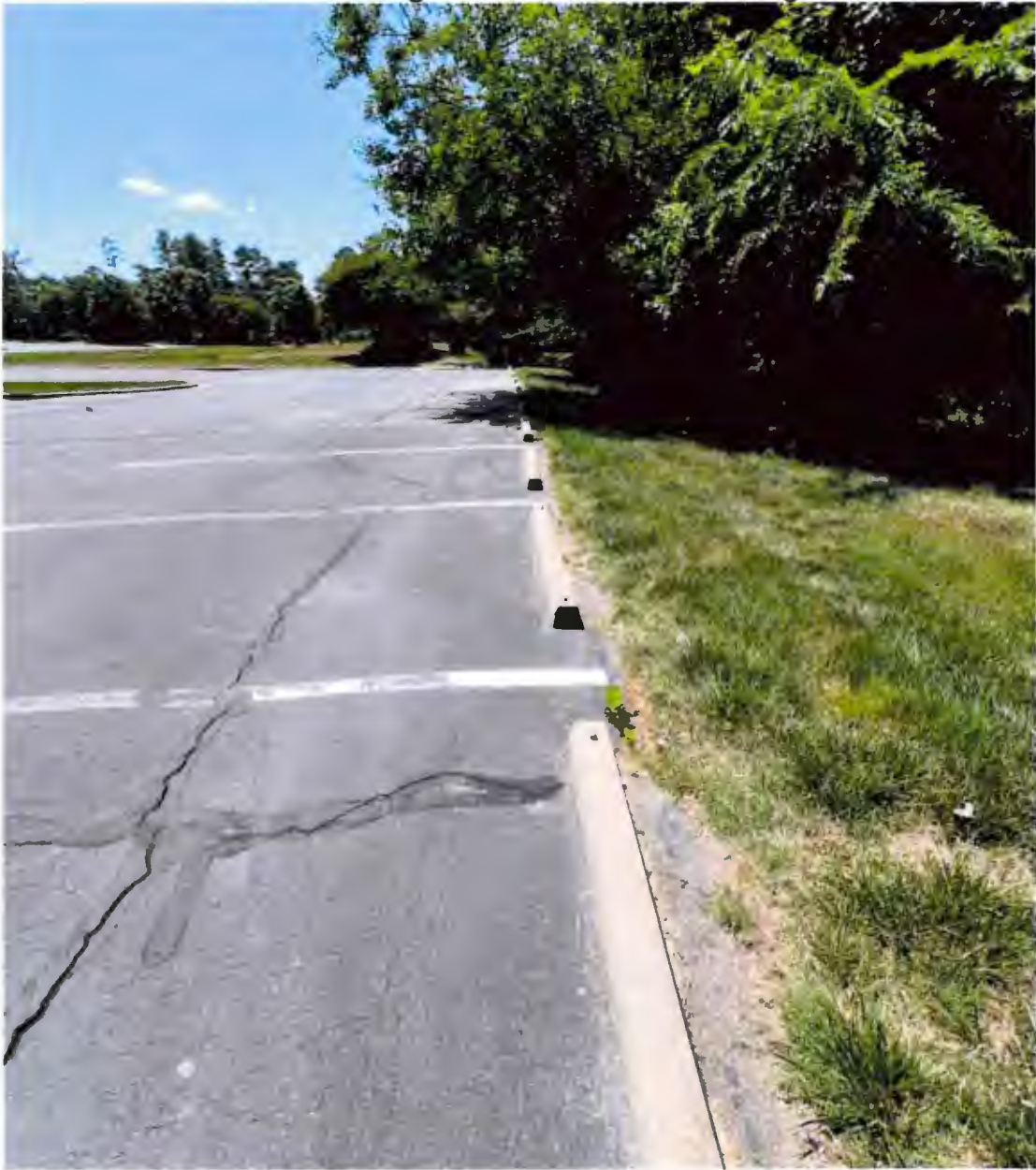
Pavement drains to pond.
