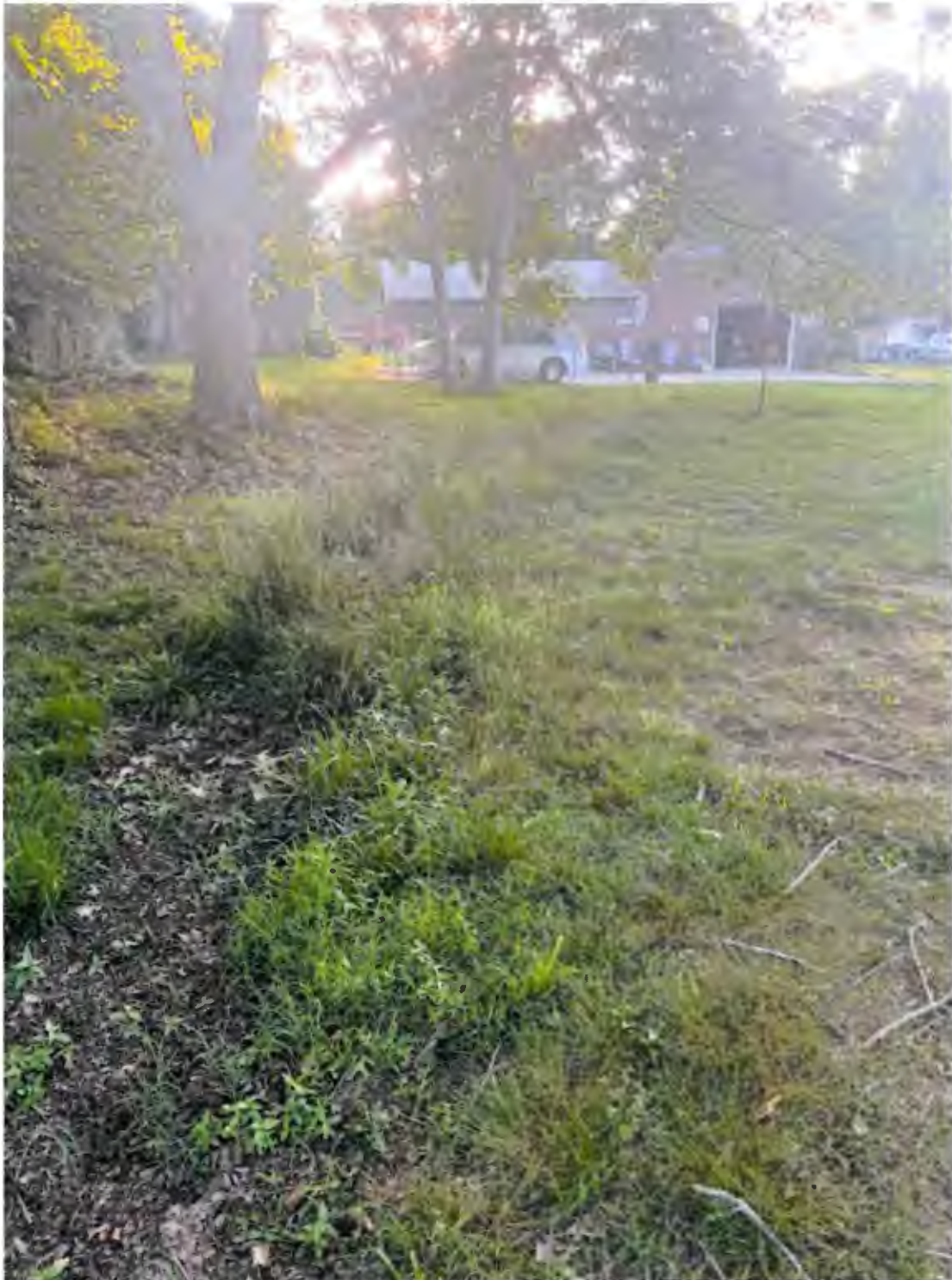
Swale has settled and is lower than the end of the swale creating water to pond.
