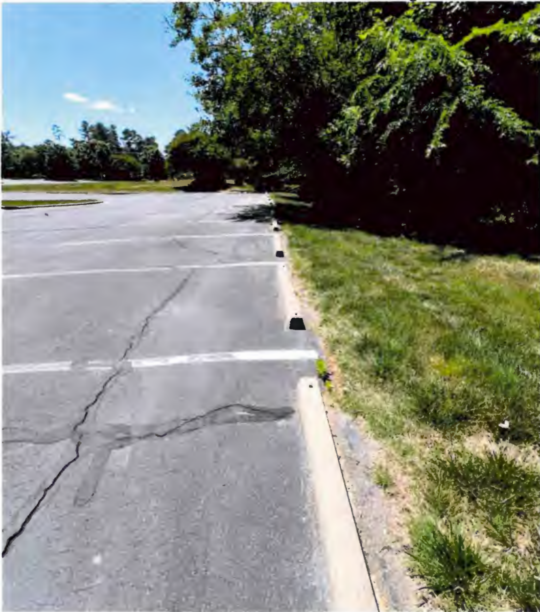
Pavement drains to pond.
