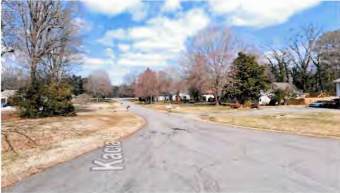
Kacia Ct. is lower than Grandover Pkwy. Some yards are lower than ditches in Kacia Ct.
